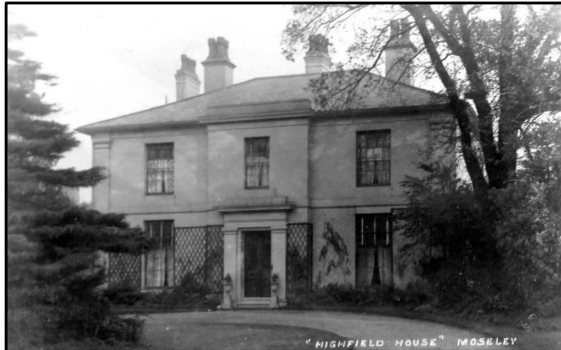
Fig.4.1: Highfield House, Church Road, c.1900. 4
