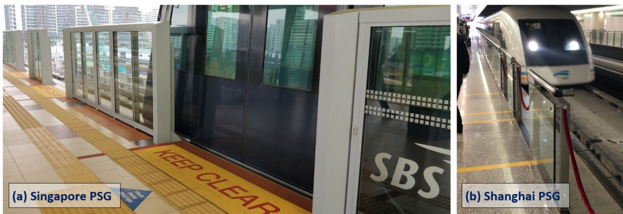
FIGURE C.1: Platform Safety Gates on [a] Singapore LRT (Author) and [b] Shanghai Maglev (Jack, 2018)
