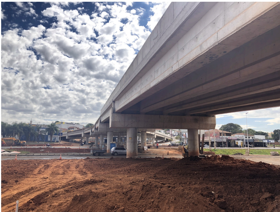
Fig. 1. “Mirassolandia” precast concrete bridge in Sao Jose do Rio Preto, SP, Brazil (reproduced with permission of www.migliorepastore.com.br ).
