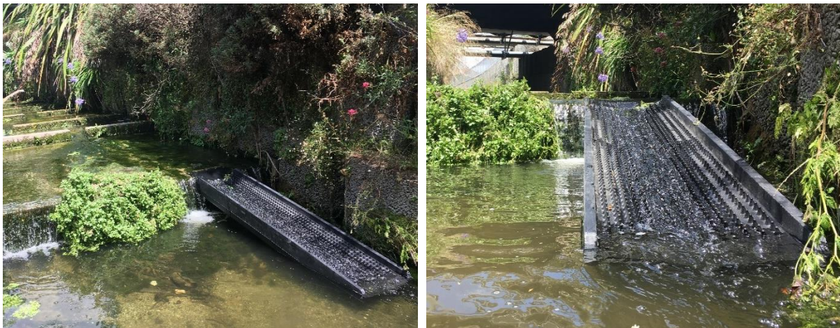
Figure 5.1. Plastic fish ramp, lined with small cusps, similar to the one used in Fake (2018), installed onto the vertical drop of the bridge apron along the Mangarau stream.
