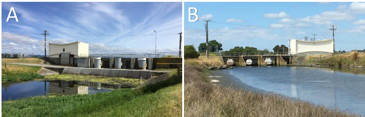
Figure 7.99. A pumping station divides the upstream and downstream sites along the Purimu Stream. A: Front view showing the structure's three jockey pumps and weed/ trash screen. B: Rear view showing its three closed discharge culverts.
