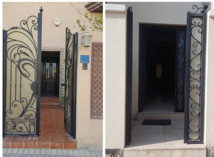
Figure 9. Inner door facing the exterior door.
