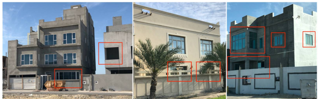
Figure 7. Openings on the ground floor are exposed to exteriors.
