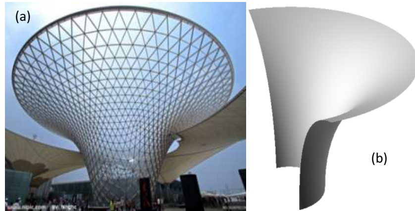
Fig. 29. Sun Valley in Shanghai World Expo Park: (a) perspective view and (b) NURBS surface.
