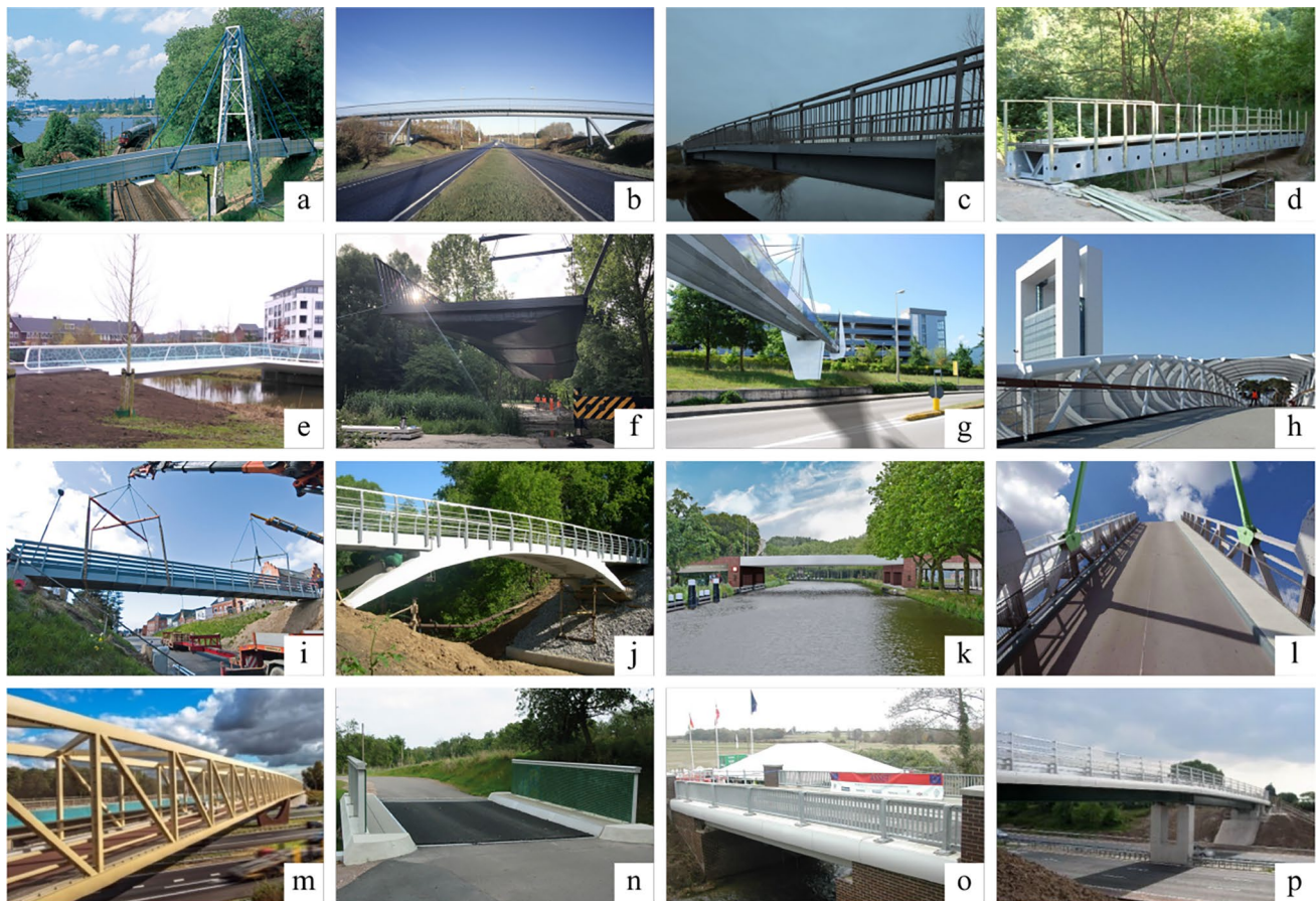
Fig. 4 Applications of composite material in bridges. a–j pedestrian bridges. k–p Road bridges. locations: Kolding, Denmark ( a ), Svendborg, Denmark ( b ), Esbjerg, Denmark ( c ), Grosseto, Italy ( d ), Harderwijk, Netherland ( e ), Rotterdam, Netherlands ( f ), Univer-
