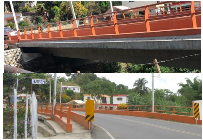
Fig. 3 El Cacique Bridge; bridge deck and access ramp
