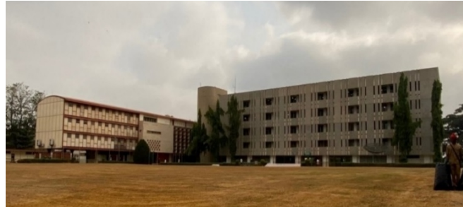
Figure 2—Old library block (constructed in 1959) on the left side, facing north and naturally ventilated; and the new library block (opened in 2001) on the right side, facing west and equipped with ACs
