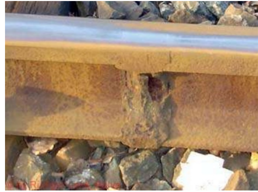
(b) Typical welded rail joint (Zwolski, 2012)
