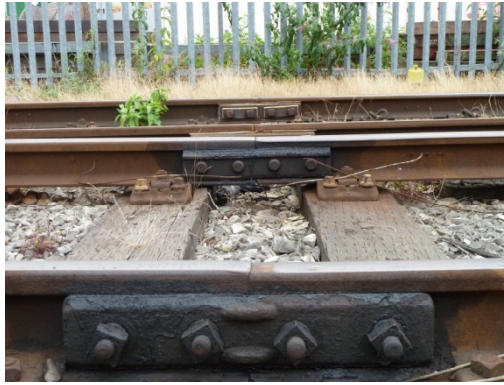
(a) Typical fishplated rail joint (Interflon, 2011)
