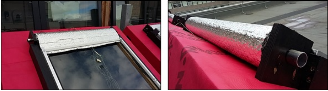
Figure 3.19: Night cover – aluminium foil bubble insulation secured to a roller blind and held in place, once rolled down, by aluminium channels
