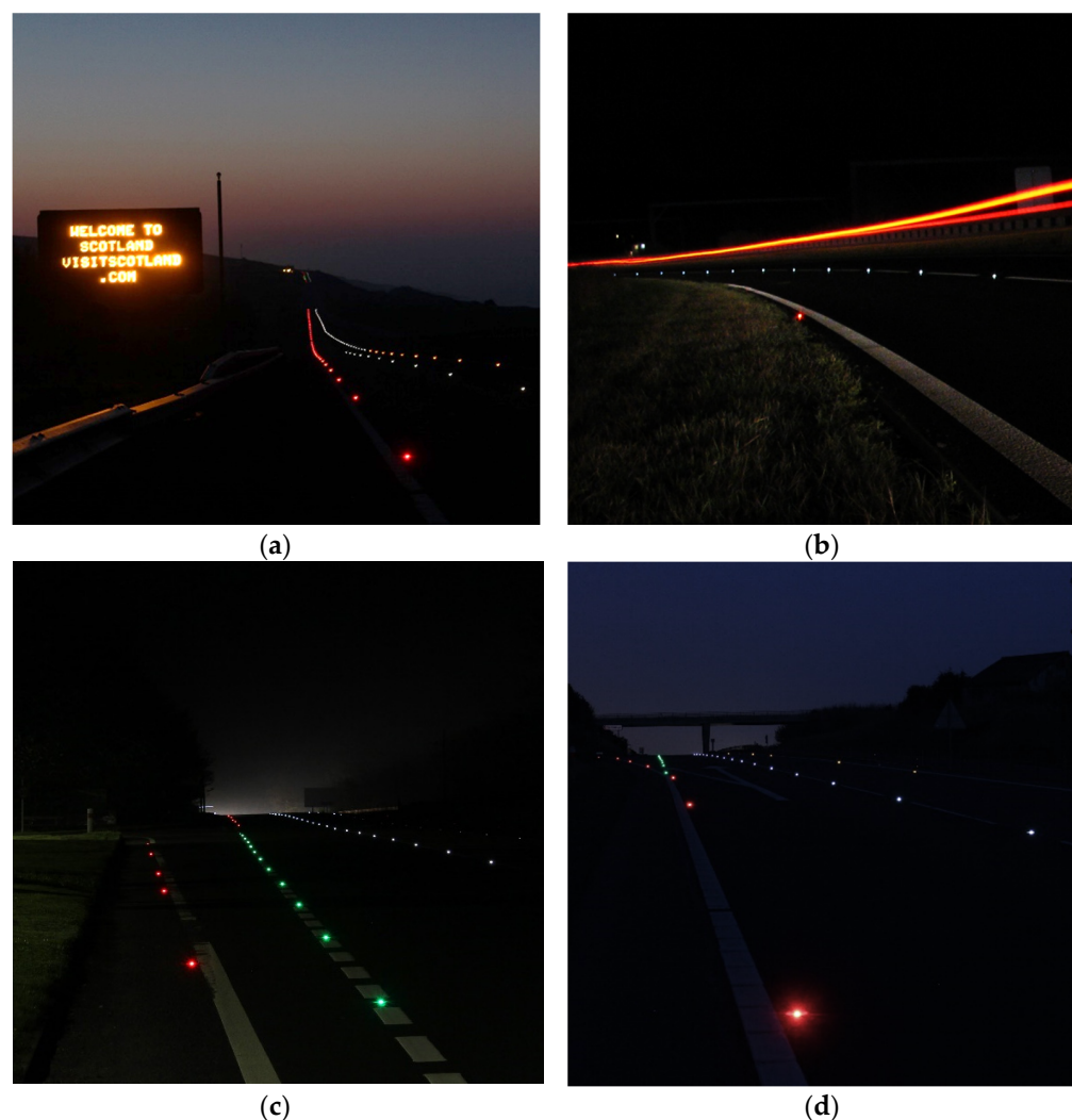
Figure 1. Example active stud installations: (a) dual to single carriageway merge; (b) single carriageway curve; (c) single carriageway junction; (d) dual carriageway junction.
