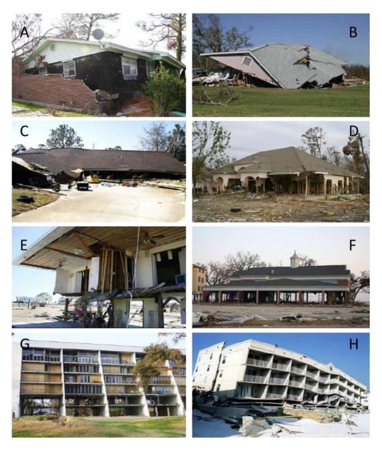
Figure 9.5 Examples of previous US storm surge damage to buildings [source: Marshall (2014)]
