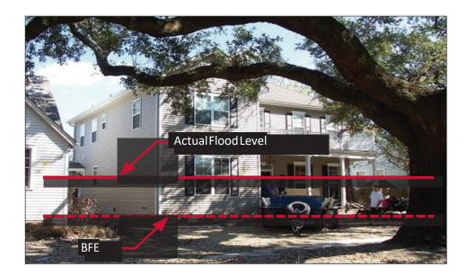
Figure 5.7 Comparison of base flood elevation level (BFE) designated by FEMA and actual flood level observed during Hurricane Katrina [source: Select Bipartisan Committee (2006)]
