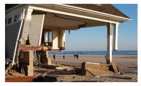
Figure 5.13 Oceanfront house in Rockaway NY, damaged during Hurricane Sandy [source: FEMA (2013)]
