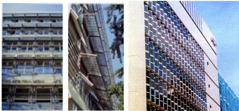
Figure 7. Fixed sunshades in the SUVA building. A commercial office building in Switzerland, built in 1993 [64]
