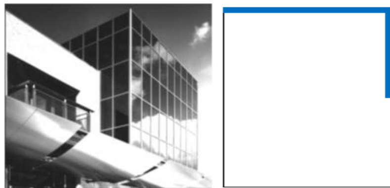
Figure 3. APS office facility in California [60]
