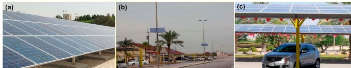
Figure 3. Selections of PV installations in Bahrain, where: (a) 0.5 MW polycrystalline solar PV installed at the University of Bahrain; (b) PV panels mounted on street lights in Alwali town; and (c) PV panels mounted on carports in Alwali town. Adapted from [20].
