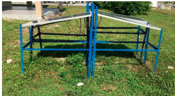
Figure 3. The front view of the photovoltaic (PV) panel arrangement at the G3 building in UTM, KL.
