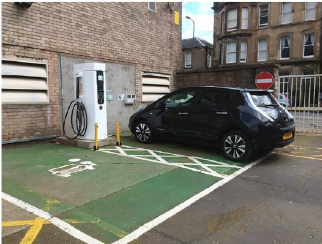
Figure 135 - Rapid charger CHAdeMO at Napier University. (Plugshare 2016)
