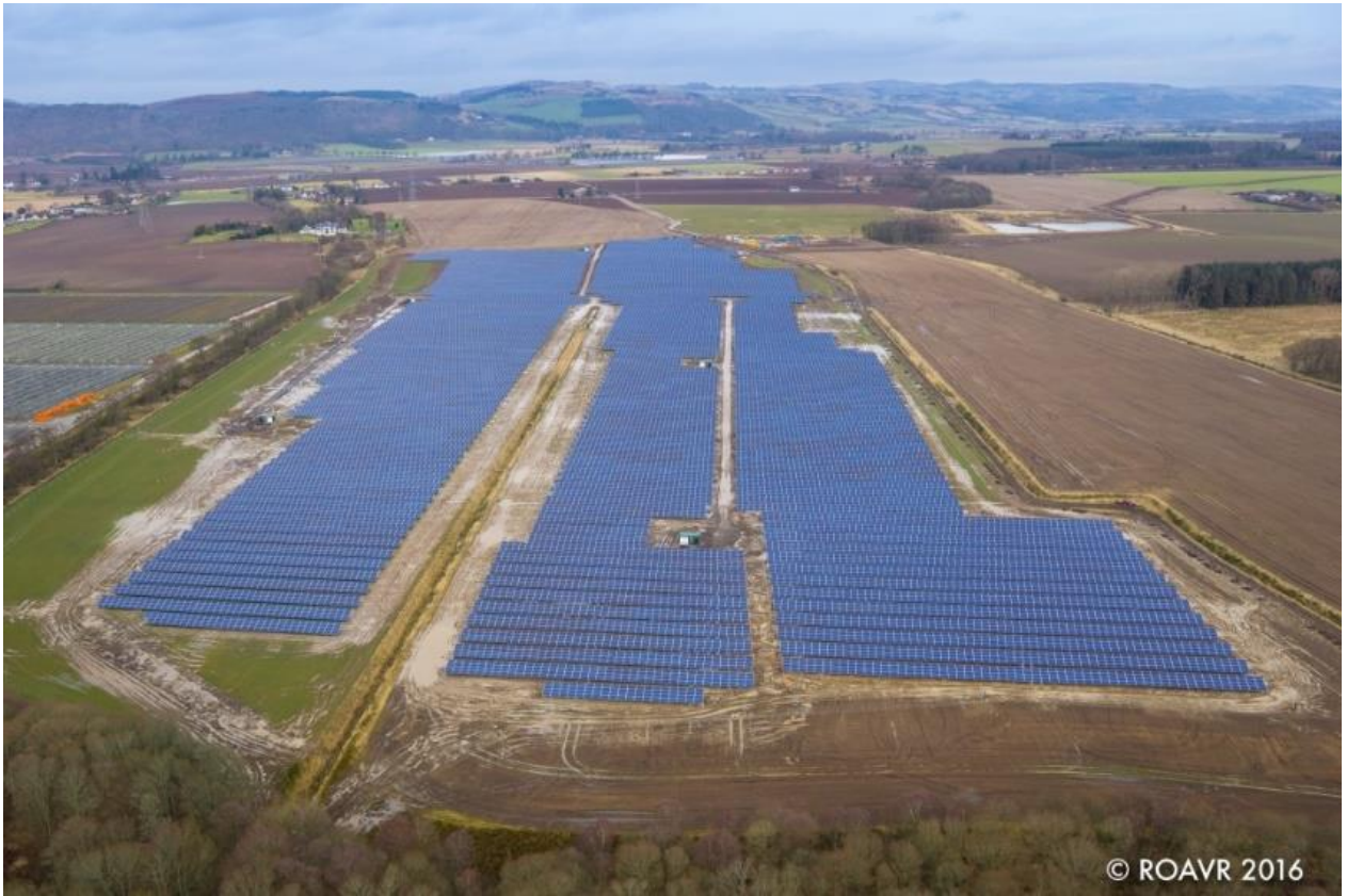
Figure 4 Errol Estate Solar Farm (Source: ROAVR 2016)
