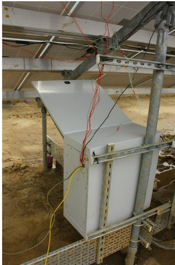
Figure 47 Data-Logger Housing
