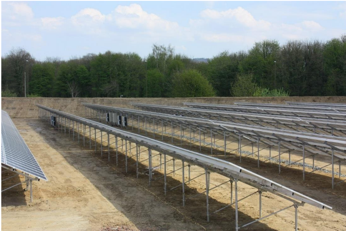
Figure 25 View from W of Site (back of panels)
