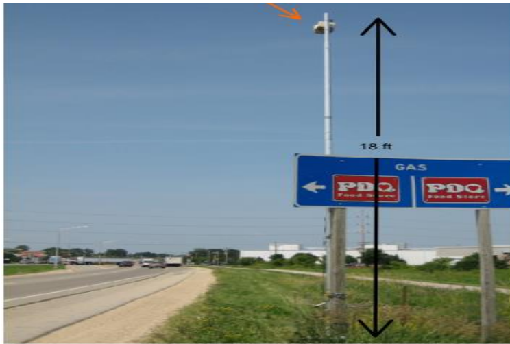
Figure 2-2: Typical analog video camera mounted on signpost overlooking the intersection to record traffic flow (Source: Gates et al., 2007)
