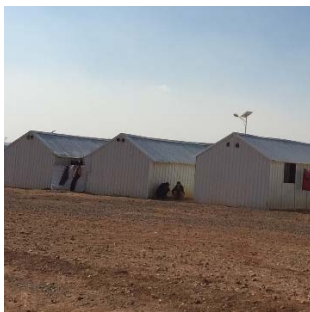
Fig. 21 Original gap between shelters [15]
