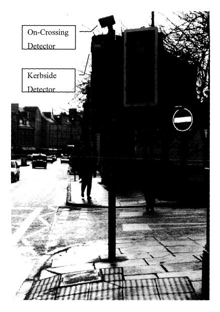
**Figure 2**: Signal pole equipment of a Puffin crossing. The centre of the figure shows the invitation to cross signal (red/green man) mounted so as to clarify its role as being an invitation to start to cross. The two detection units can be seen mounted at the top on the signal pole, one pointing down over the kerbside and the other left onto the crossing area.
