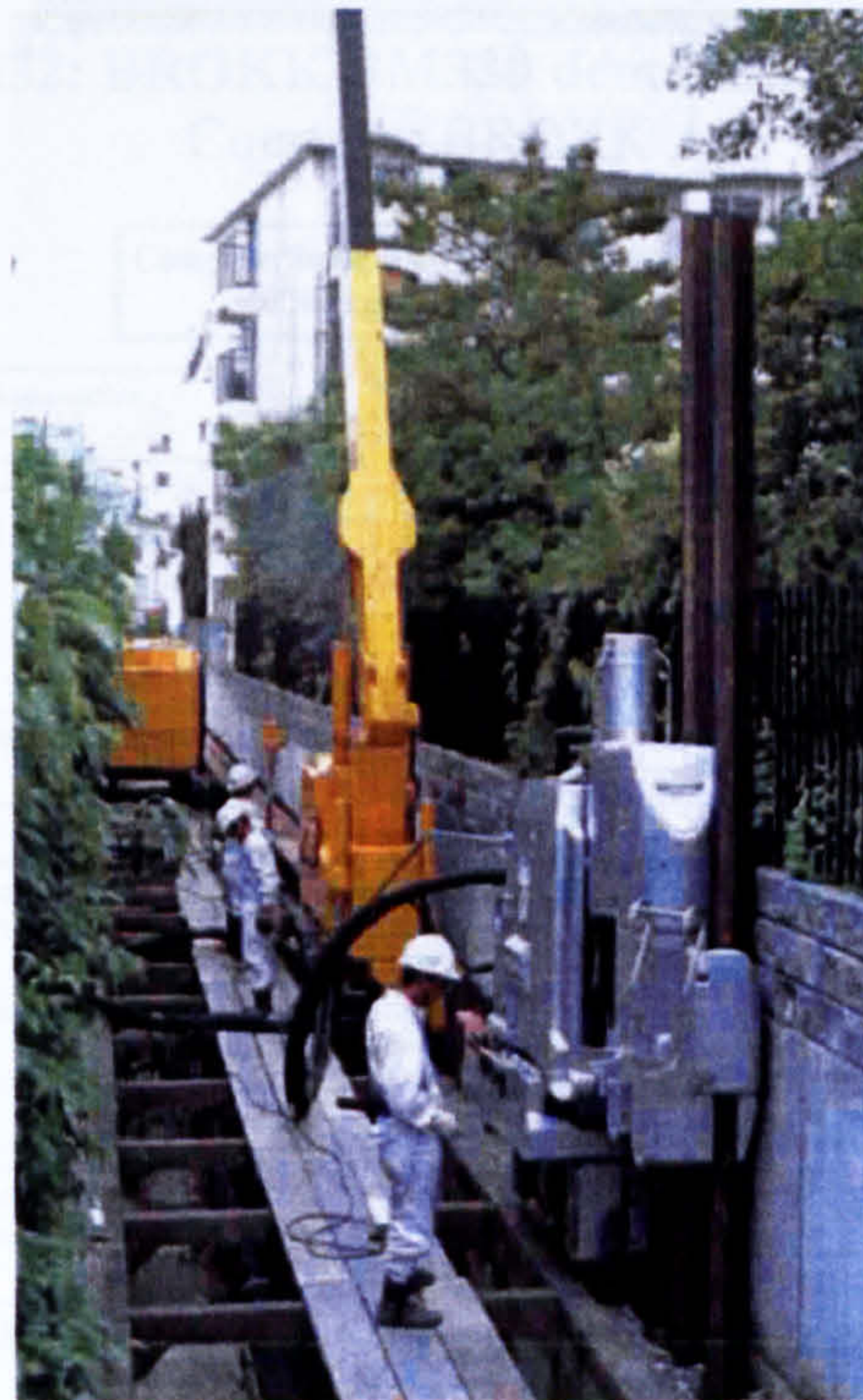
Figure 3.31: Automatic pile installation system Courtesy: Giken Seisakusho Co. Ltd.
