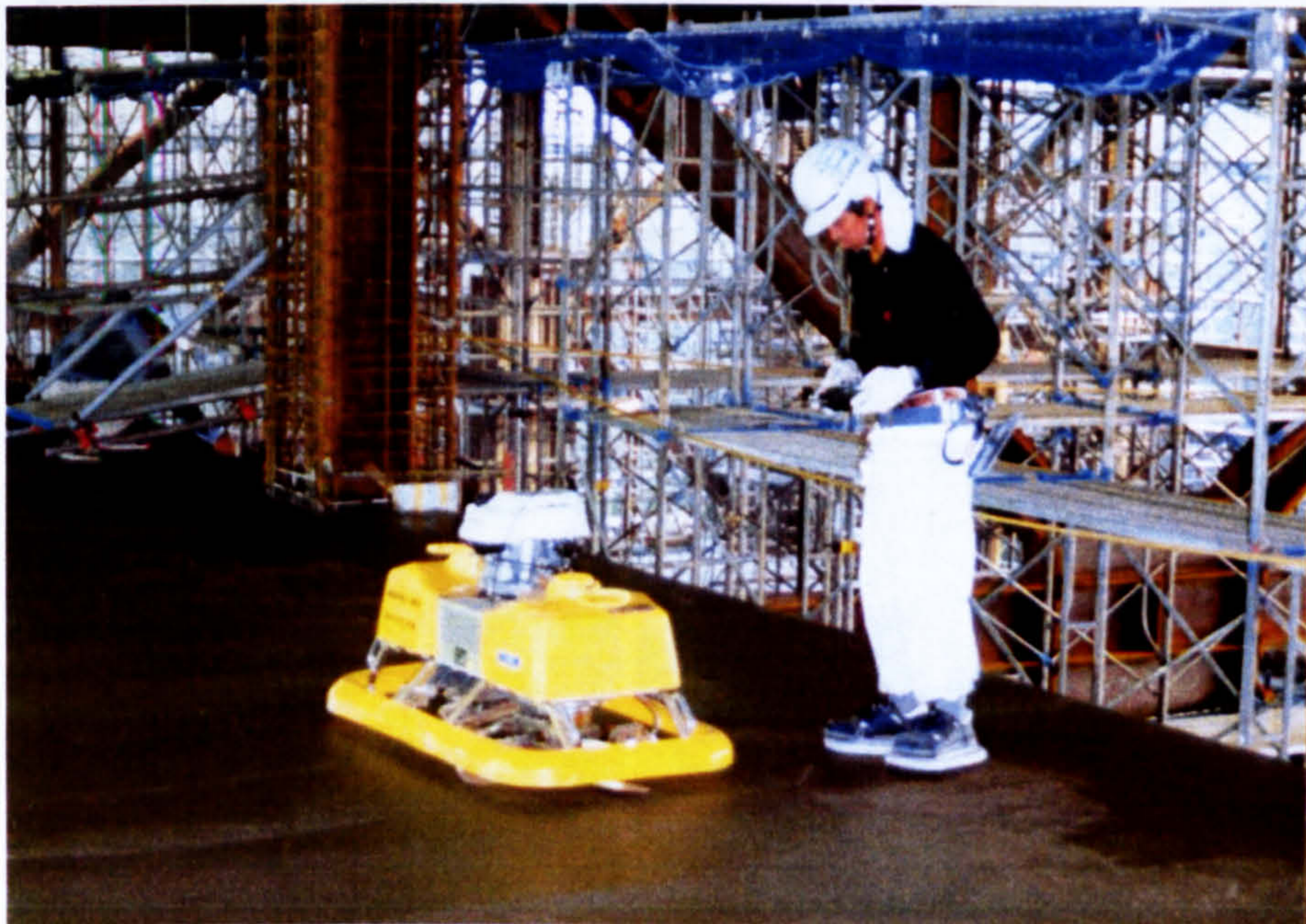
Figure 3.11: Robocon, tele-operated concrete trowelling system Courtesy: Tokimec Construction Systems Inc & Takahashi Construction Systems Inc.
