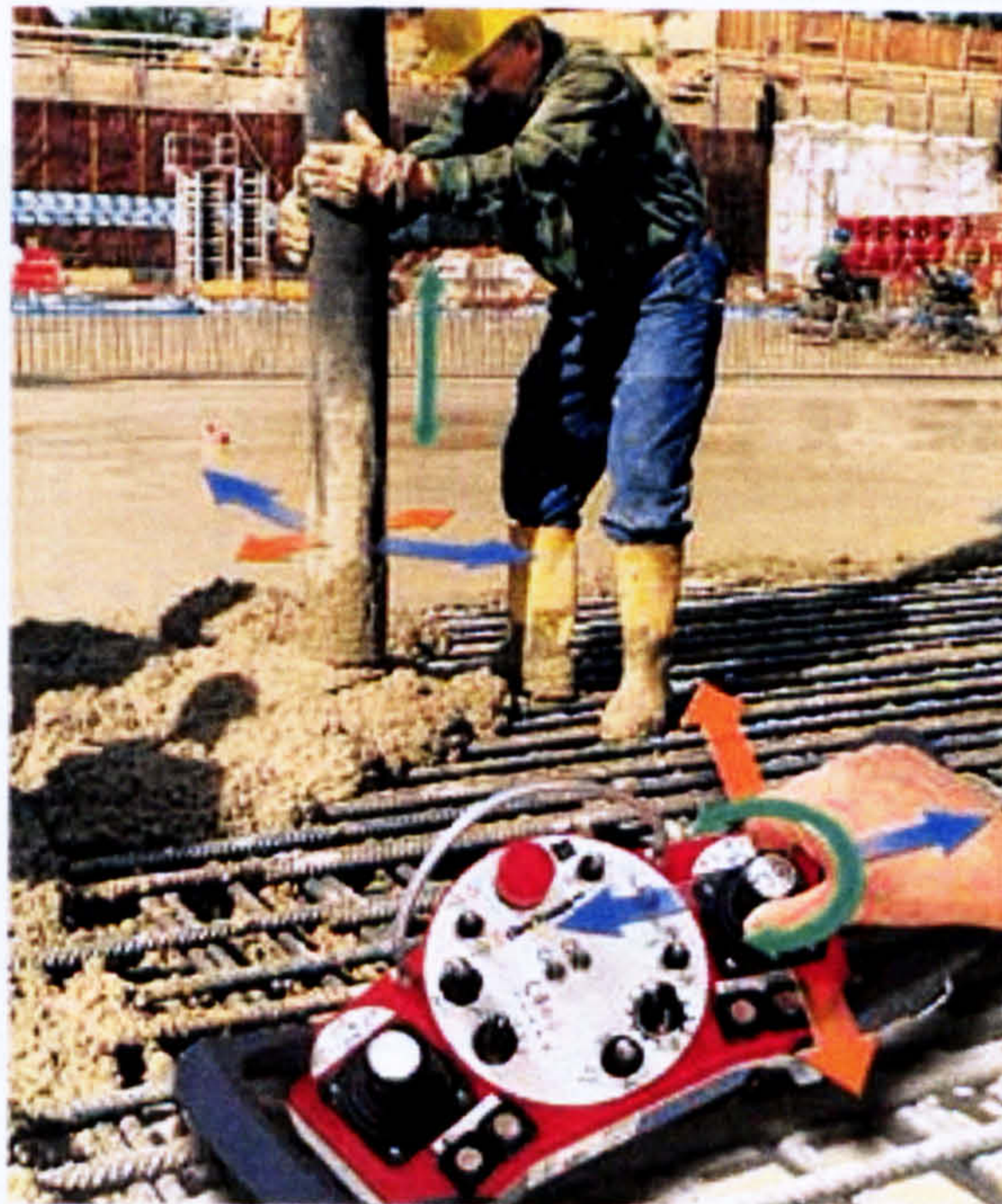
Figure 3.9: Tele-operated concrete boom pump Courtesy: Putzmeister UK Ltd
