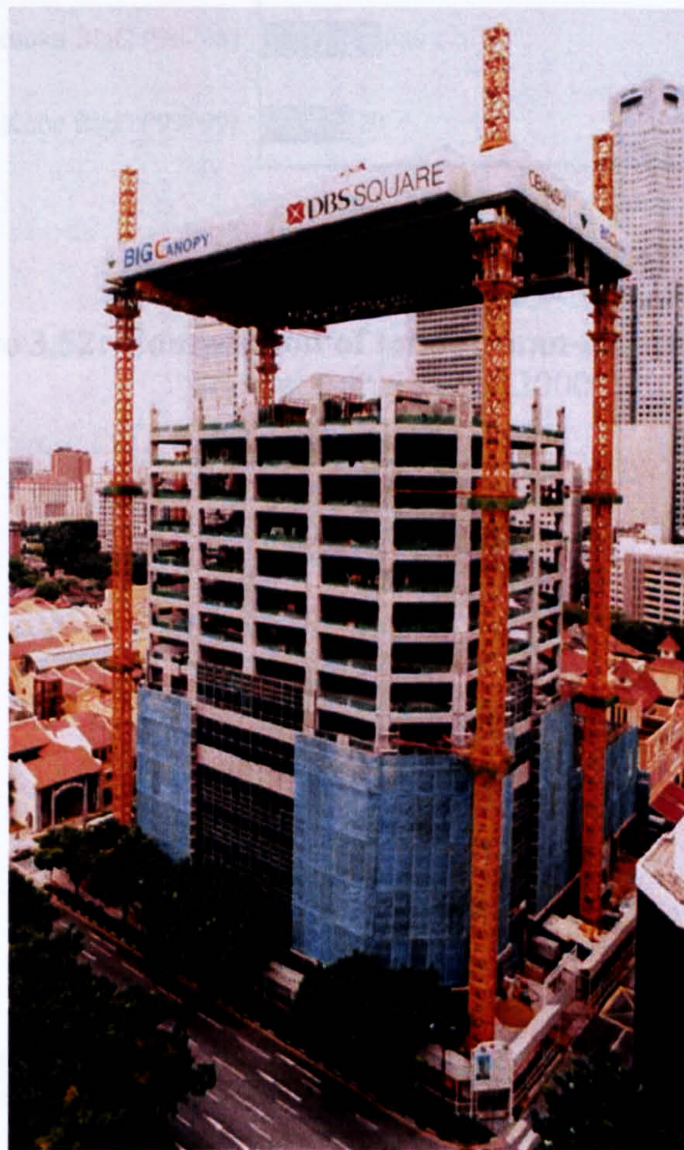
Figure 3.51: Big-Canopy high-rise construction system, DBS Square, Singapore Courtesy: Obayashi Corporation
