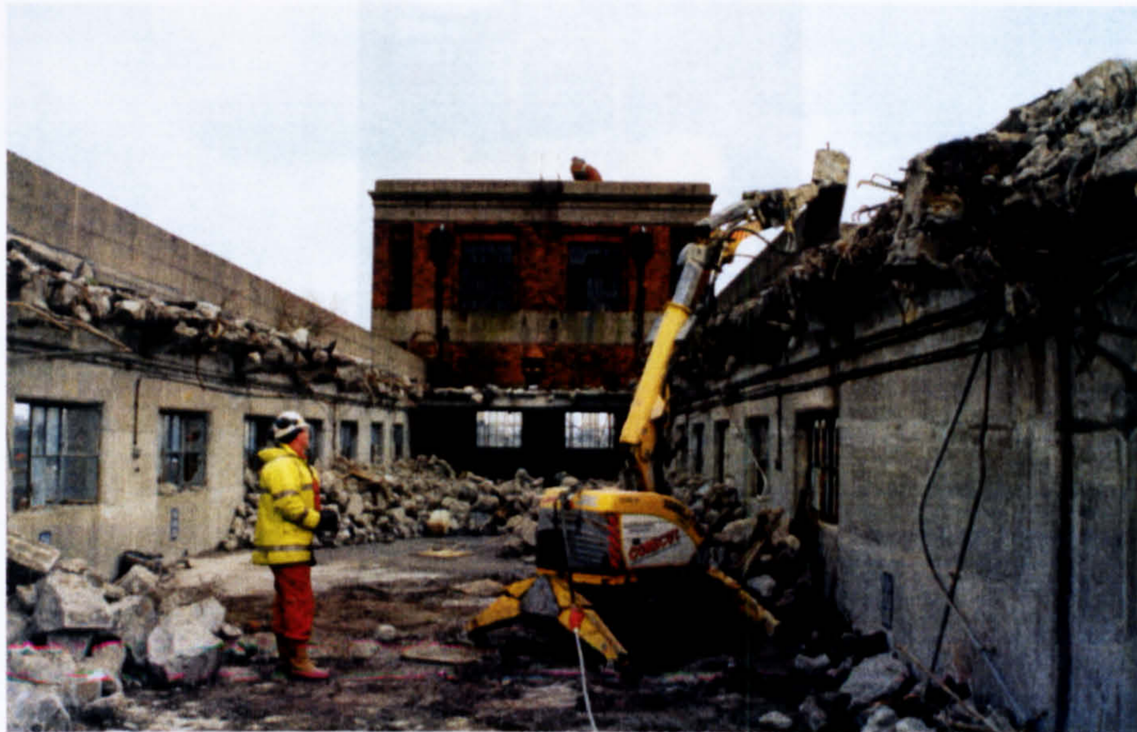
Figure 3.54: BROKK BM150, Meadowside Granary demolition project Courtesy: Corecut Ltd & Scotdem Ltd
