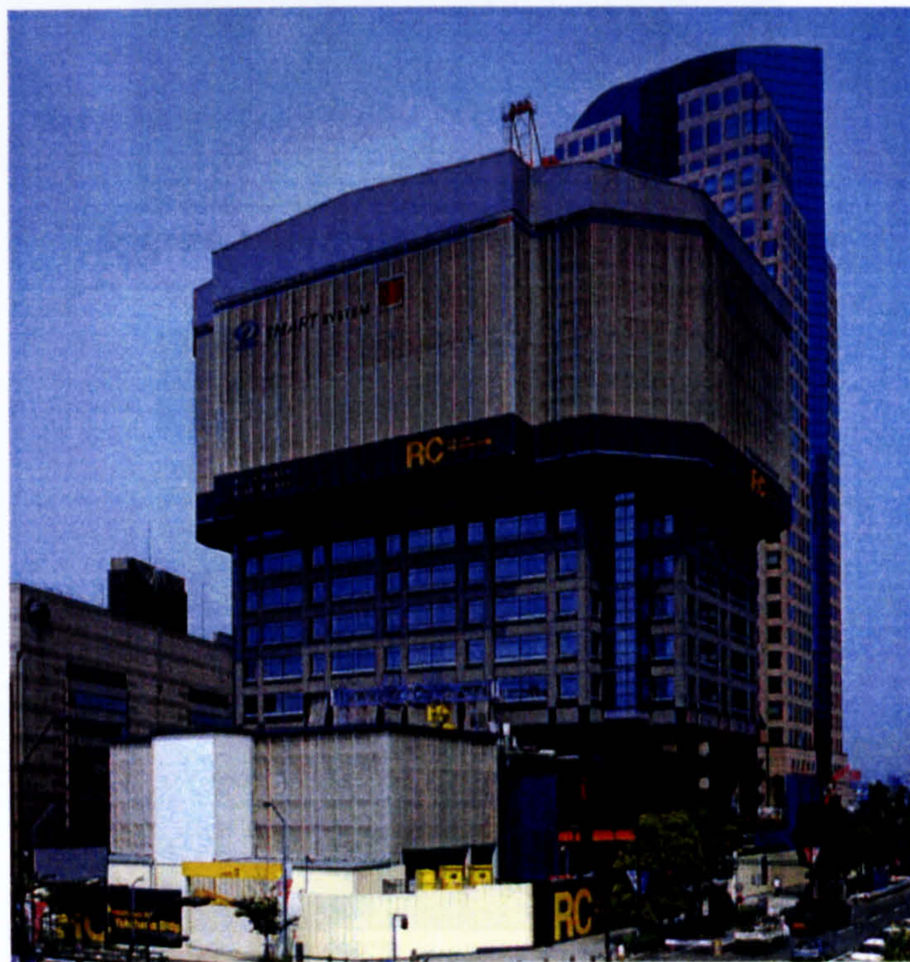
Figure 3.35: SMART system exterior view, Juroku Bank, Nagoya Courtesy: Shimizu Corporation
