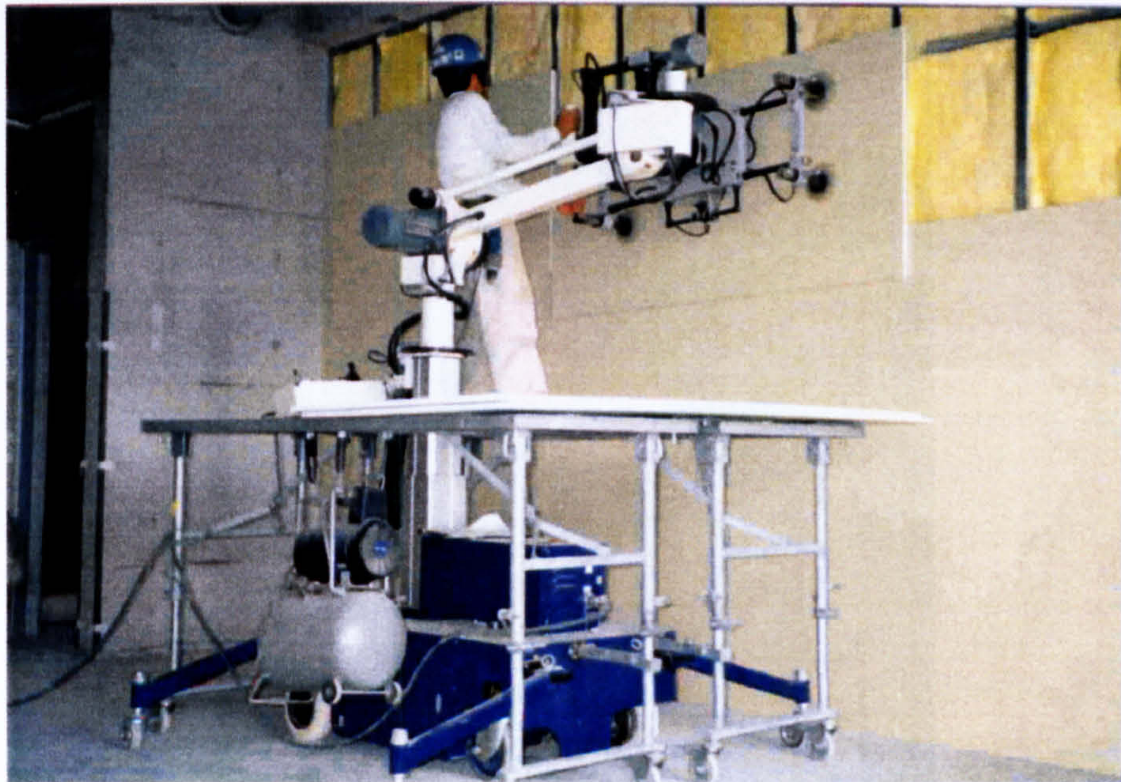
Figure 3.13: Lightweight material manipulator Courtesy: Tokyu Construction Co. Ltd.
