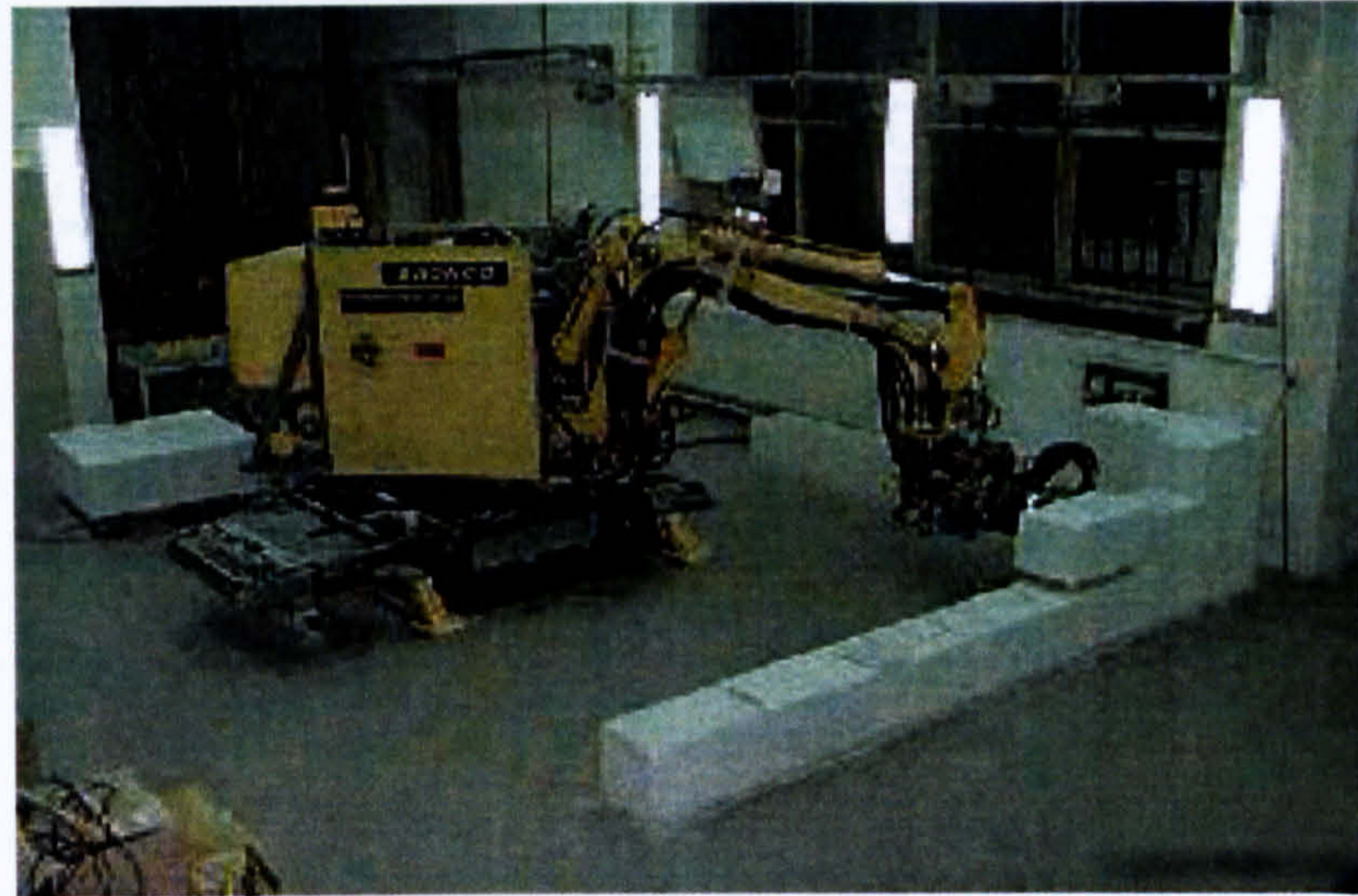
Figure 3.26: BRONCO, automated masonry construction system Courtesy: University of Stuttgart, ISW
