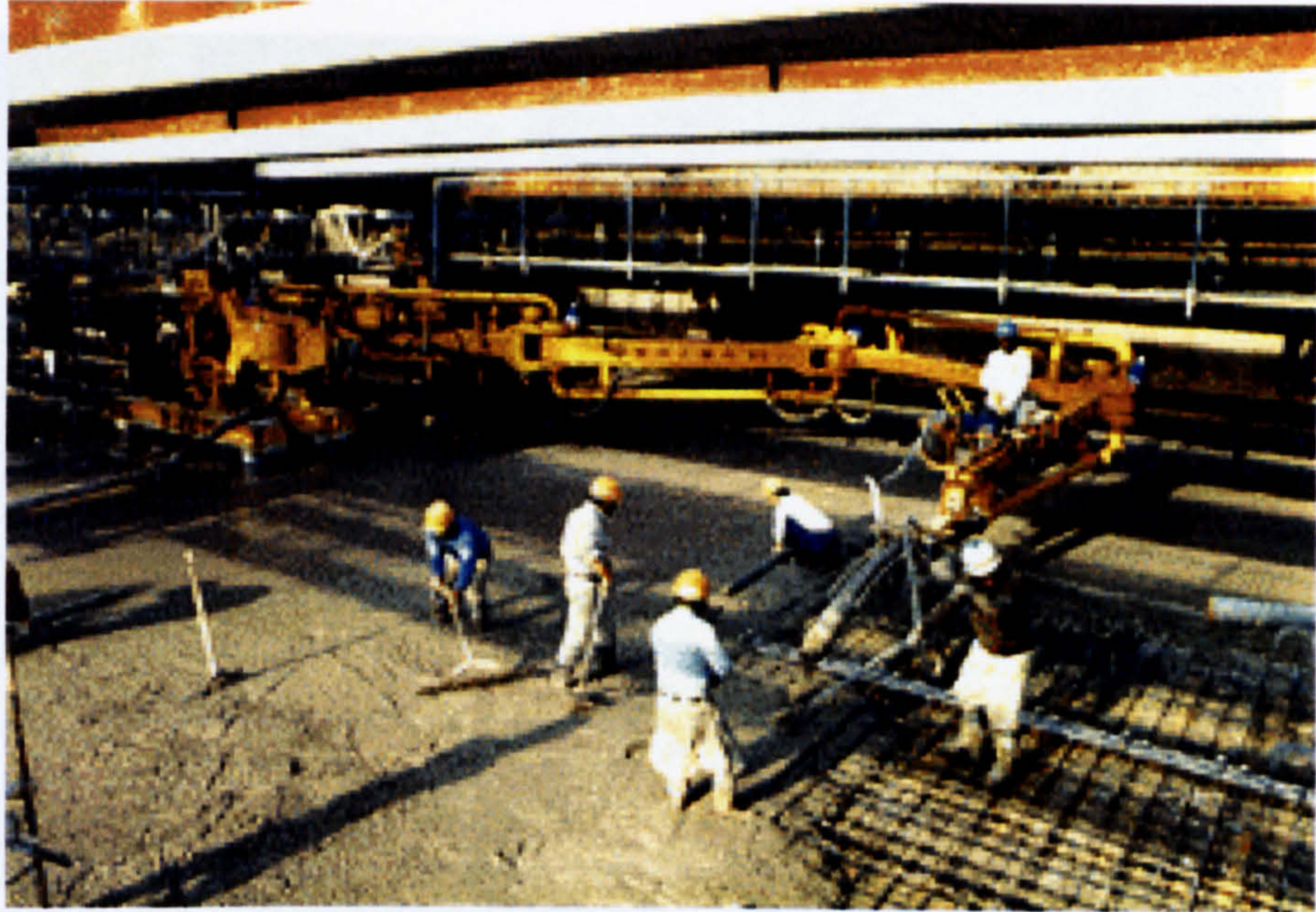
Figure 3.8: Horizontal concrete distributor Courtesy: Takanaka Corporation
