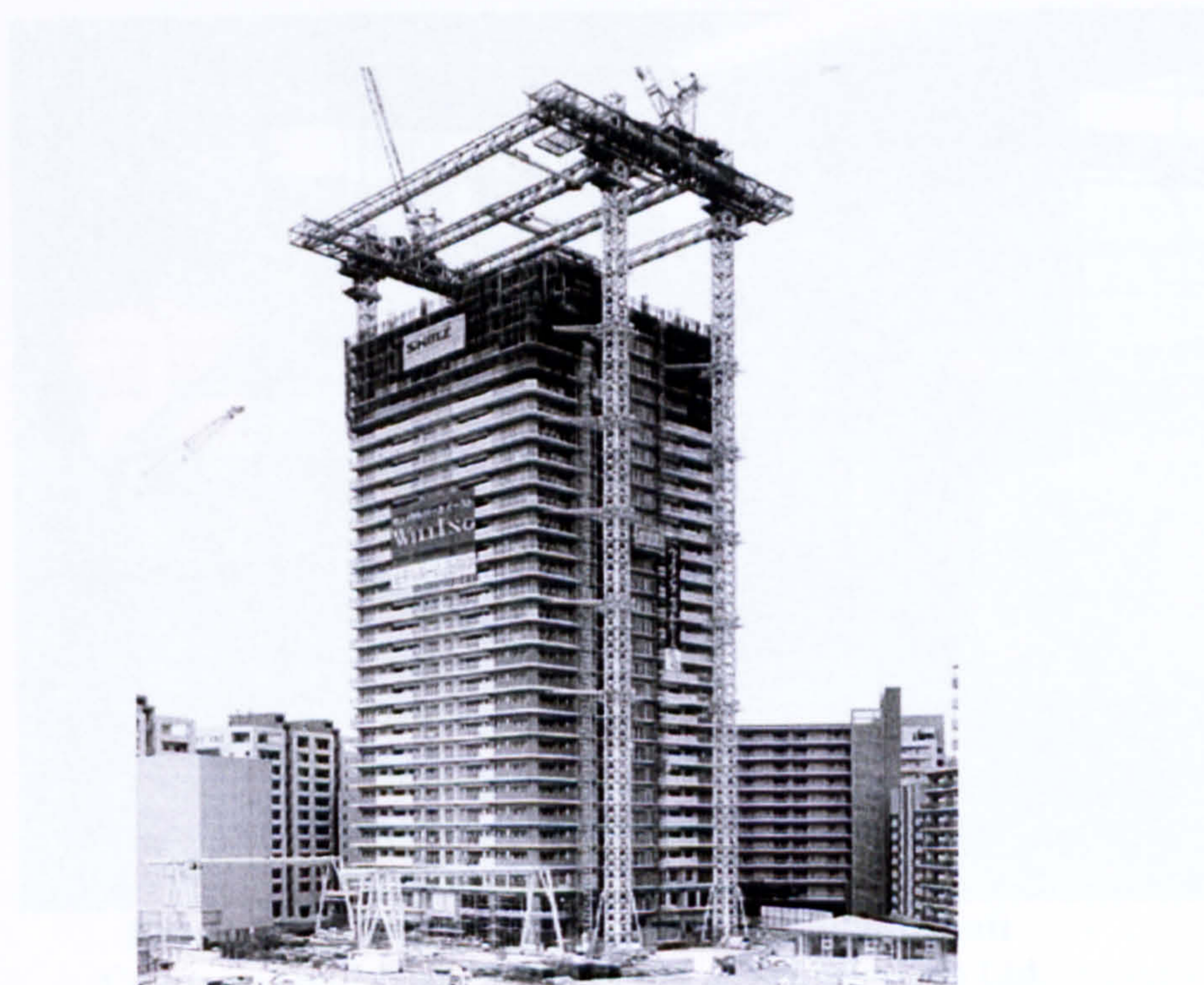
Figure 3.53: New SMART system, Central Park West Sea Tower project Courtesy: Shimizu Corporation
