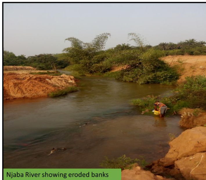
Figure A-9-4 Njaba River showing exposed soil banks and gully erosion cracks Source: Author's fieldwork
