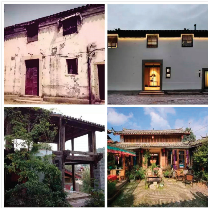
Figure 3. Refurbishing Old Rural Houses in Lijiang. Source: the pictures are collection from ‘100 rural house refurbishing cases’, retrieved from http://www.360doc.com/content/16/0819/17/33281137_584378177.shtml .
