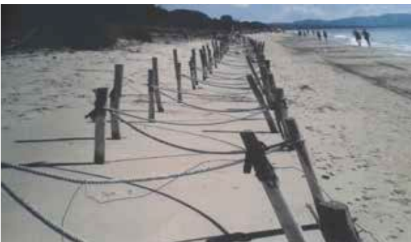
Figure 7 - The sticks and piles of logs tied by a rope were dispersed in the sea by the storms.
