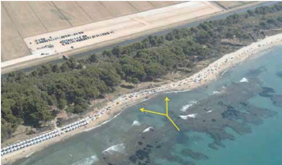
Figure 2 - Flat beach-rocks dampen the impact force of the waves that arrive at the beach. Where there are breaks in the rocks erosion has changed the beach (yellow arrows).
