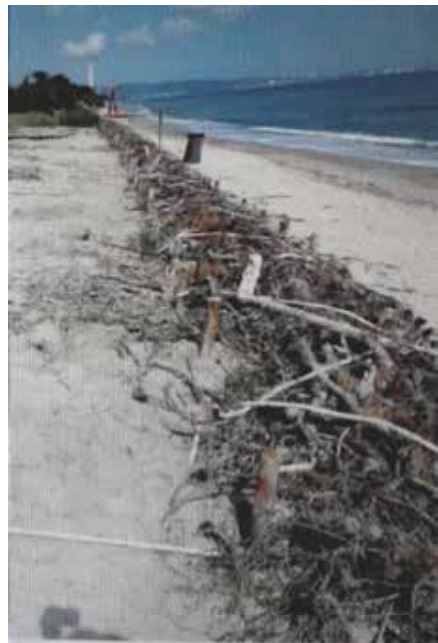
Figure 4 - Sticks and piles of logs tied by a rope.
