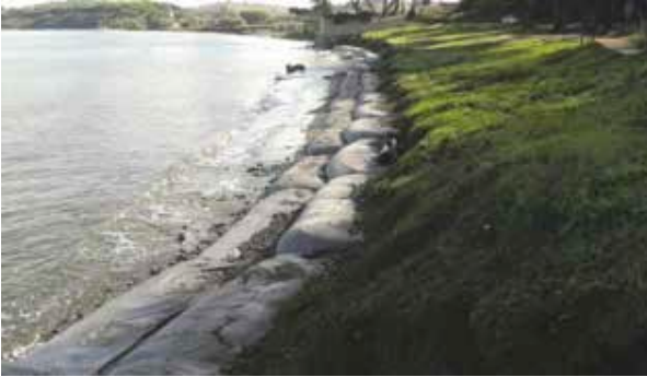
Figure 5 - Sacks of geotextile cloth containing sand.
