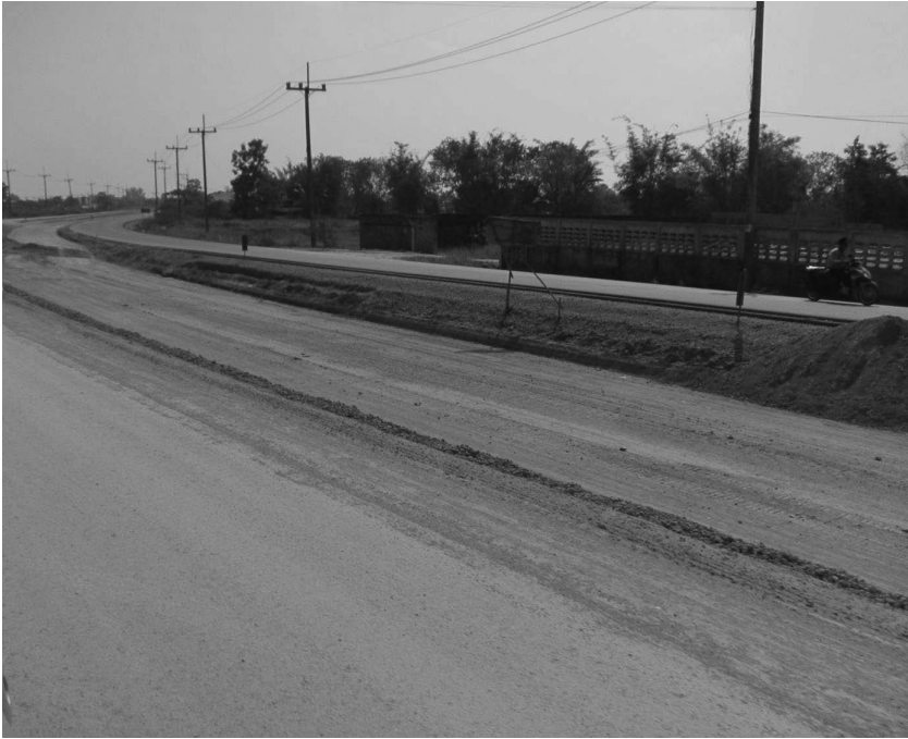
Figure 8.5 Road expansion in Mae Sai
