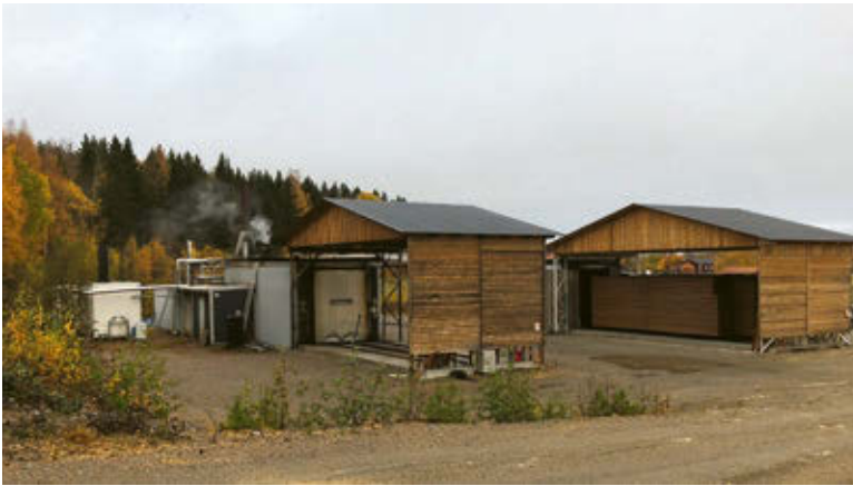
Figure 16: Example of a small scale thermal modification plant (ThermoWood)
