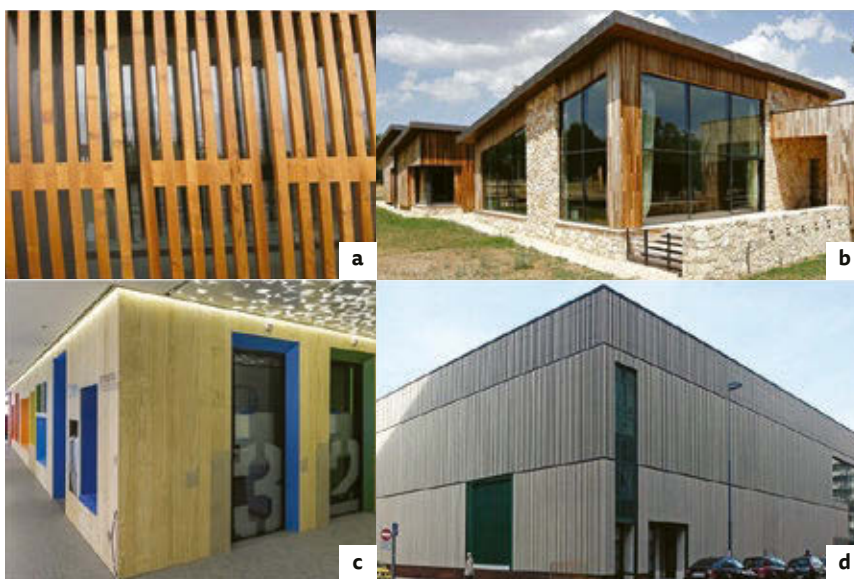
Figure 40: Examples of the use of modified wood: a) Façade of thermally modified Radiata pine, Madrid, b) façade of thermally modified Eucalyptus, Segovia, c) Accoya interior panels, Google office Madrid, and d) Accoya façade, congress palace Vitoria
