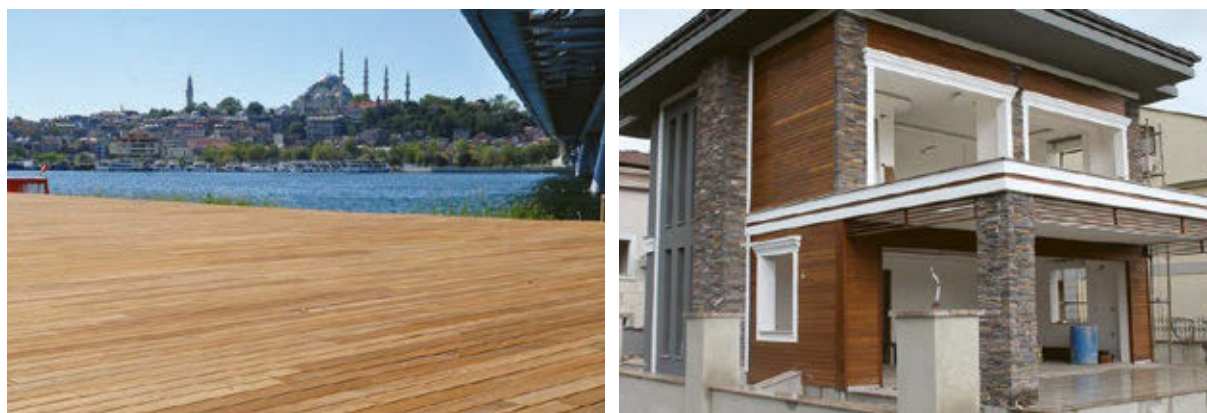
Figure 44: Examples of the use of modified wood: thermally modified wood decking (left), and thermally modified iroko wood cladding (right)
