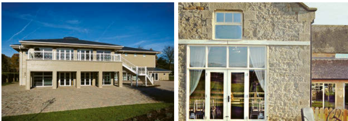
Figure 46: Accoya cladding at Pipers High School London (left), and the joinery company Richard James in Northumberland, UK
