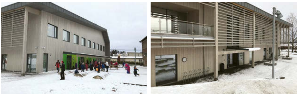
Figure 33: Chemically modified radiata pine cladding (Accoya). Lislebyhallen, Fredrikstad, Norway. Photo: Ostfold Research/Lars Tellnes
