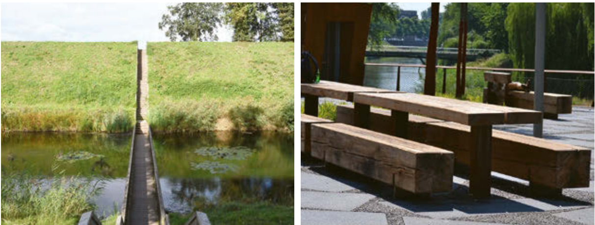
Figure 29: Accoya sunken pedestrian "Moses" bridge (left), and FirmoLin extreme dimensioned TM Douglas fir (right)
