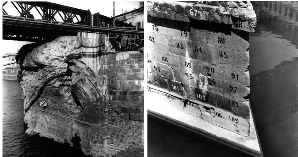
Fig. C-23. Left: The ruin of one of the piers of the Ponte a Santa Trinita: note the temporary Bailey bridge placed over the remaining piers by the Allies soon after the war. Right: The various parts of a remaining pier were numbered before being dismantled (Gizdulich Archive, Florence, reproduced from Belli).
