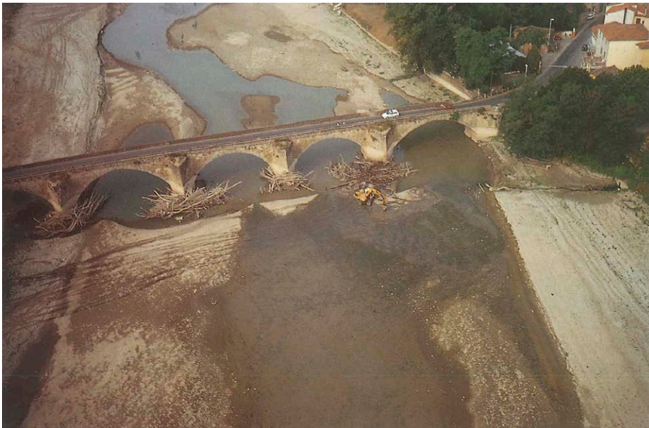
Fig. 3-9. The Buriano Bridge connects the banks of the Arno River along the Cassia Vetus, the old road which connected Rome to Florence, crossing Arezzo. It may possibly incorporate a preexisting Roman bridge. Buriano Bridge and Ponte Vecchio are the only historical bridges remaining along the course of the Arno River. The heightening of La Penna dam would lead to its submergence for less than 24 hours during exceptional floods (recurrence time of the order of a century) (Reproduced from 1996 Hydraulic Risk Plan).
