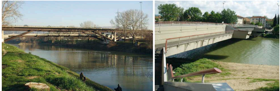
Fig. C-14. The Varlungo bridge (left) and the Giovanni da Verrazzano bridge (right).
