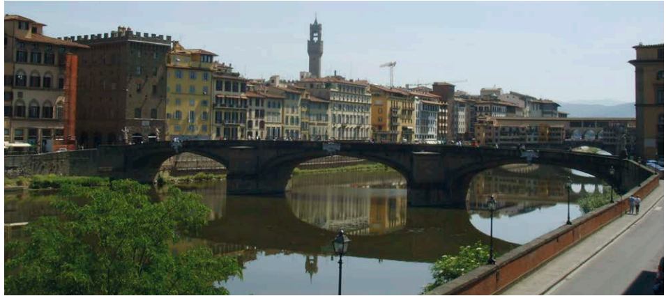
Fig. C-25. Santa Trinita bridge today. View from Palazzo Bardi Guicciardini's terrace.
