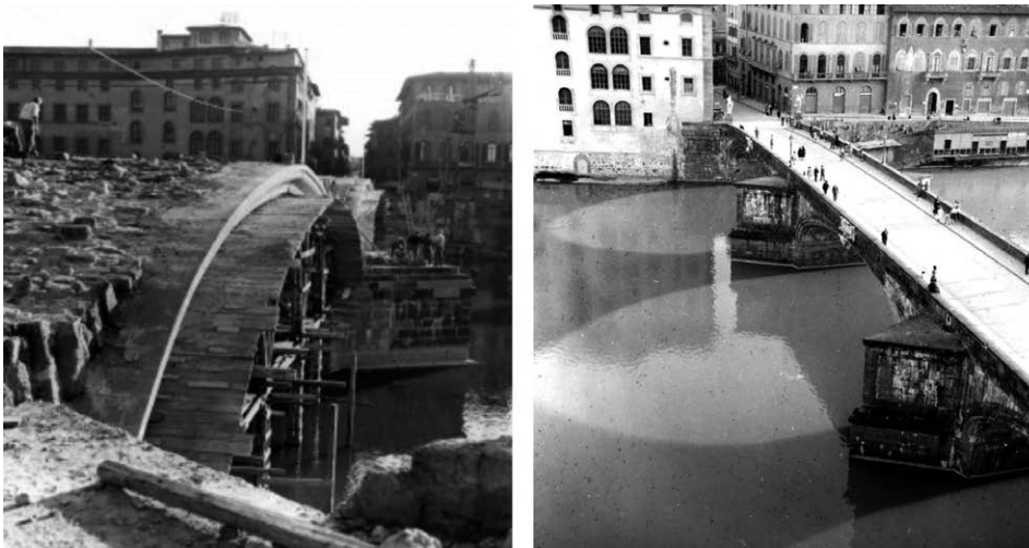
Fig. C-24. Left: The Ponte a Santa Trinita during the reconstruction of the central arch, 1956; Right: The bridge just after its completion, 1958 (Gizdulich Archive, Florence, reproduced from Belli).
