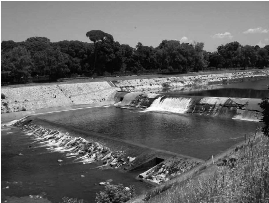
Fig. C-12. The Isolotto weir and counter-weir.
