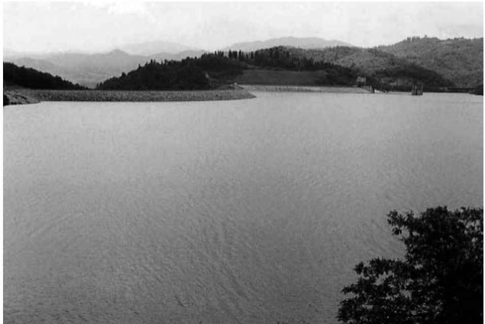
Fig. D-4. The Bilancino earthfill dam at the maximum storage (Courtesy by Dott. Grossi and Publiacqua).
