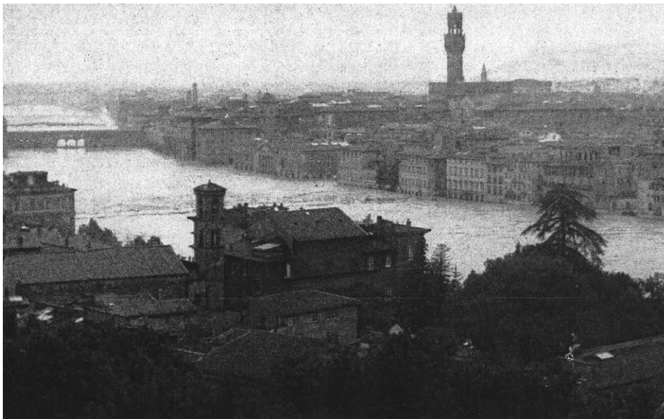
Fig. C-43. Overview of the Arno River showing Florence bridges during the 4 November 1966 flood: note in the foreground the Ponte alle Grazie that was completely submerged (Photo Caldini, reproduced from Principe and Sica, 1967).
