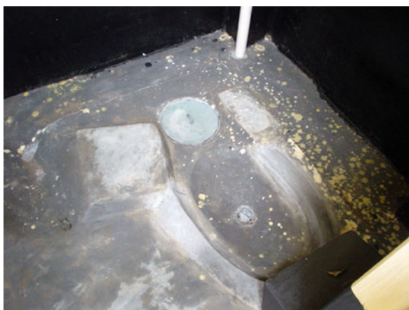
Fig. 12.6 A UDDT with double fecal chambers and anal cleaning space in Bangladesh. The fecal hole cover can be observed in the upper middle, and the urinal is in its lower-right part. The anal cleaning space is located at the leftmost middle in this picture
