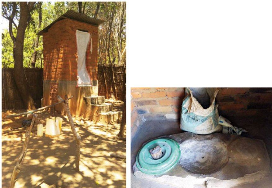
Fig. 12.4 A UDDT in Malawi: (left) outside views of a UDDT; (right) inner view of a UDDT. (The left figure was adapted from Harada and Fujii 2020)
