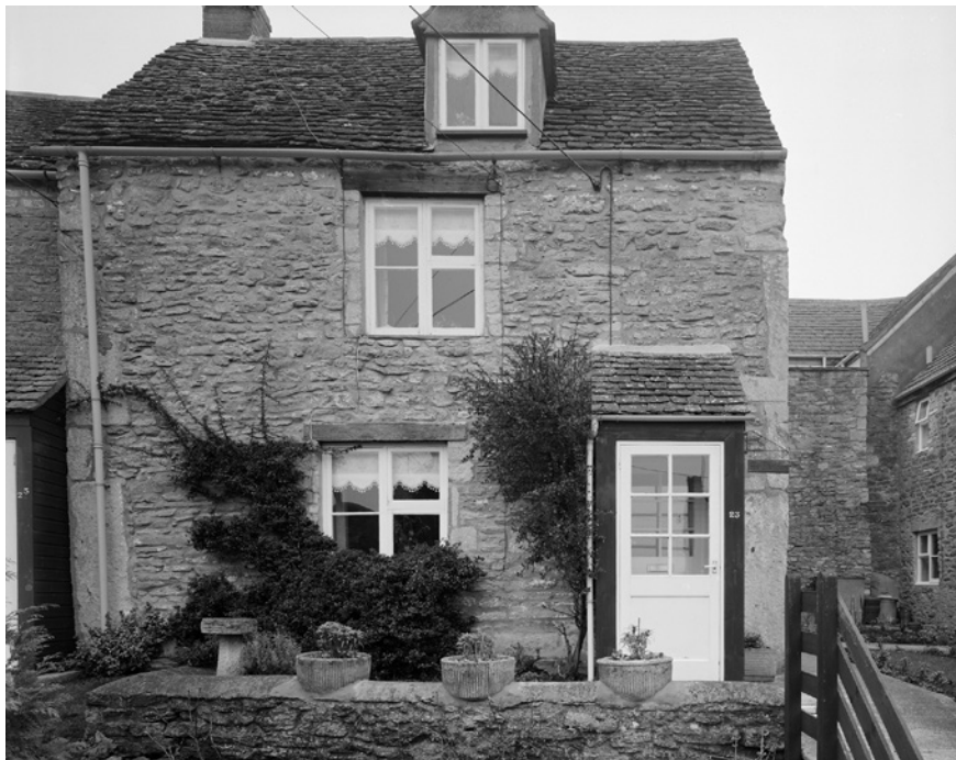
FIGURE 21.2 View of the south wall of the former chapel of St Helen at Malmesbury in 1992 © CROWN COPYRIGHT. HISTORIC ENGLAND ARCHIVE (REF. BB/15932).
