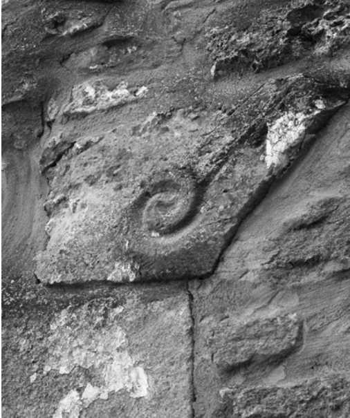
FIGURE 21.5 View of the kneeler at the top of the north-east quoin of the former chapel of St Helen at Malmesbury © AUTHOR
