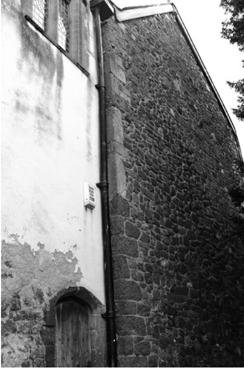
FIGURE 23.4 St Olave's church, Exeter; long-and-short quoins of primary 11th-century fabric at the west end of the nave © AUTHOR
