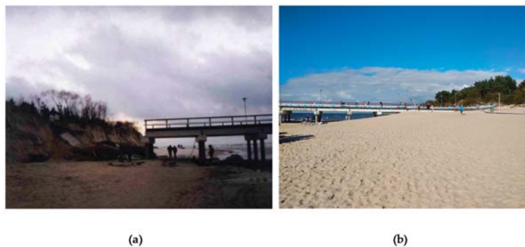
Figure 2. (a) Palanga pier after the storm “Anatol”, December 1999, and (b) in September 2018.
