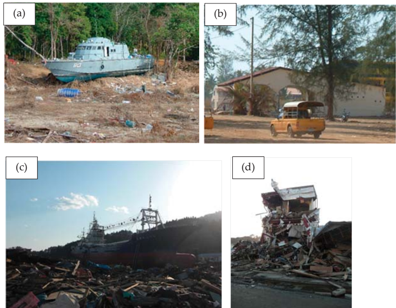
Figure 4. Damage due to ships: (a) a patrol boat stopped at the foot of a mountain located 1 km inland of Khao Lak in Thailand, (b) a building showing a big hole made by the patrol boat in Khao Lak in Thailand, (c) a large fishing boat left behind in the ruins near a fishing port at Kesennuma in Japan, and (d) a broken steel frame building that was located on the shortest line between the large fishing boat and the fishing port at Kesennuma in Japan.
