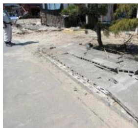
Figure 27. Block wall, inundation depth 2 m, wall fail, Kitaibaraki City.
