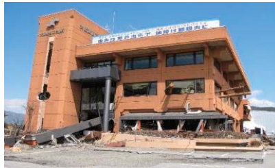
Figure 25. Reinforced concrete building, inundation depth 6.5 m, Ofunato City.
