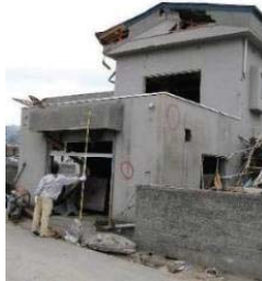
Figure 21. Reinforced concrete house, inundation depth 5.5 m, Yamada-cho.
