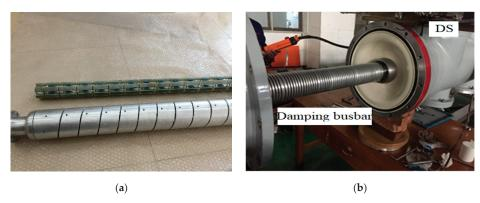
**Figure 1.** The new damping busbar installed in a gas insulated substations (GIS): (a) general view of the damping busbar with its components; (b) the placement of the damping busbar.
