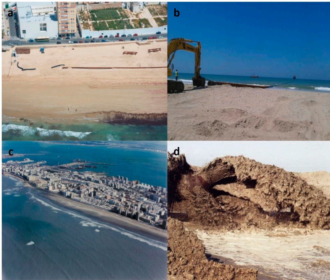
Figure 4. Different aspects of the sediment pouring on Victoria Beach, showing (a) pipe assembly; (b) transport of the pipe to the sea; (c) aerial view of the pipe while pouring; and (d) pipe outlet onto the beach.
