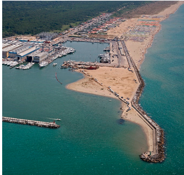
Figure 5. The updrift breakwater of Viareggio harbour and the beach close to it. Note that the sun umbrellas are far from the cabanas, bars and restaurants.
