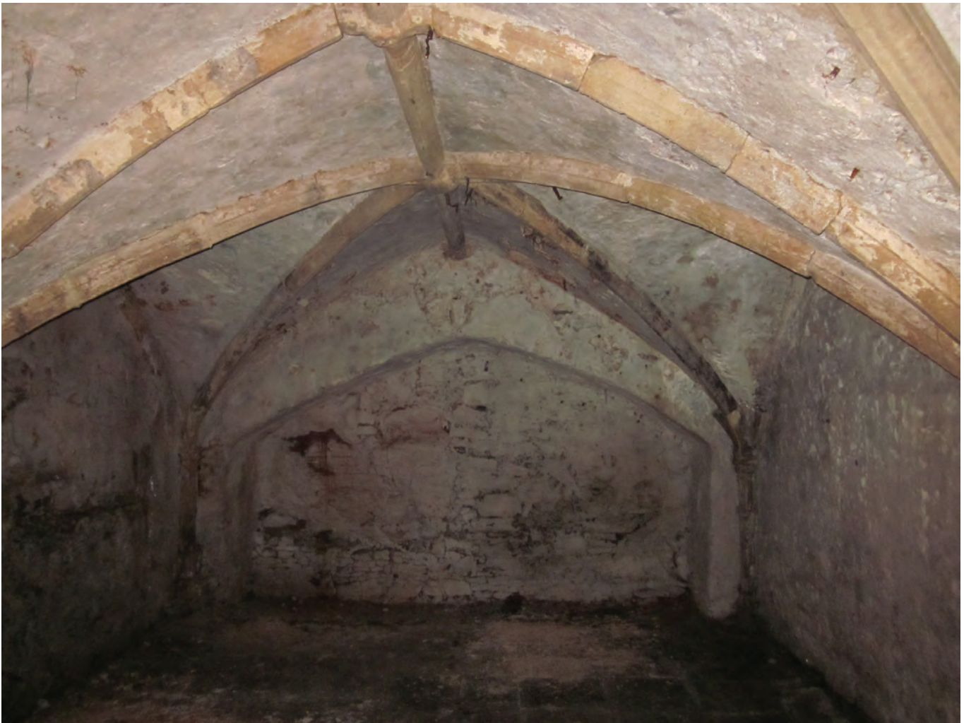
Figure 6.91 Nos 21–4 High Street. View of quadripartite vault (photograph R. Jones)
