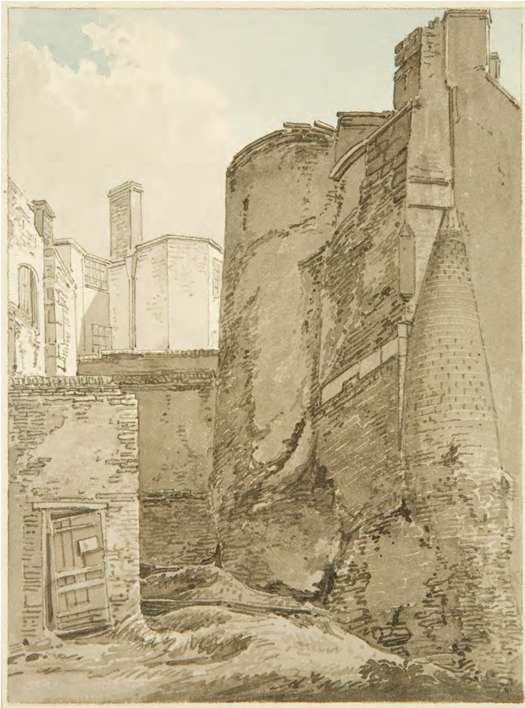
Figure 6.33 East end of New Gate during demolition in 1821 by Hugh O'Neill (Braikenridge Collection, BRSMG M2718)
