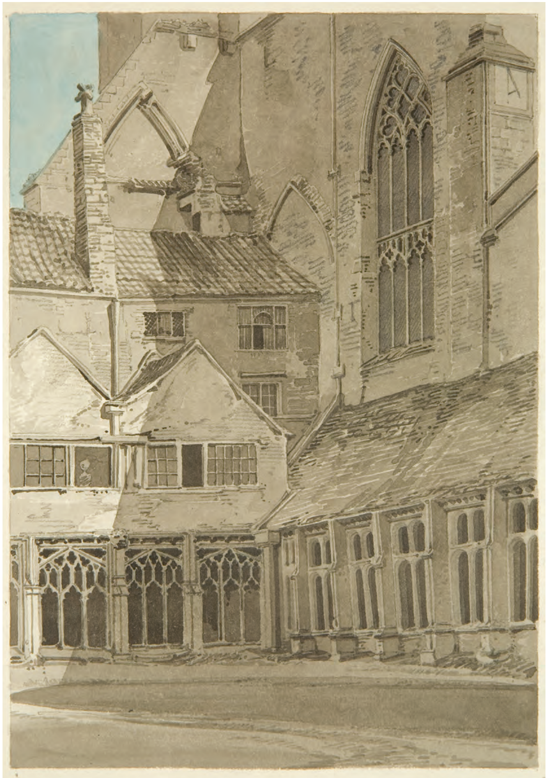
Figure 7.20 Two gabled houses on the south side of the Cathedral nave in 1821 by Hugh O'Neill (Braikenridge Collection, BRSMG M1887)
