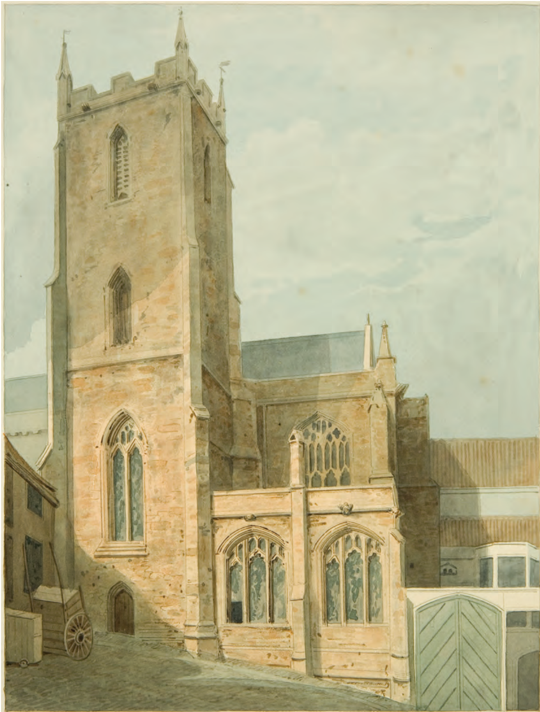
Figure 6.60 The tower and sacristy (Poynz chapel) of St Mark's Hospital from the south-east in 1825 by Samuel Jackson (Braikenridge Collection, BRSMG M2591)
