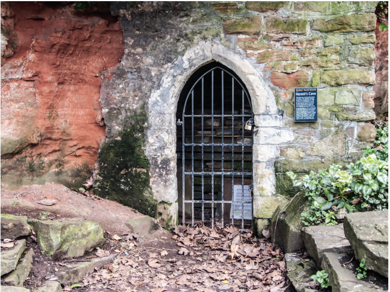
Figure 6.76 Entrance to Hermitage in Redrock Garden, part of St John's Hospital (photograph D Martyn)
