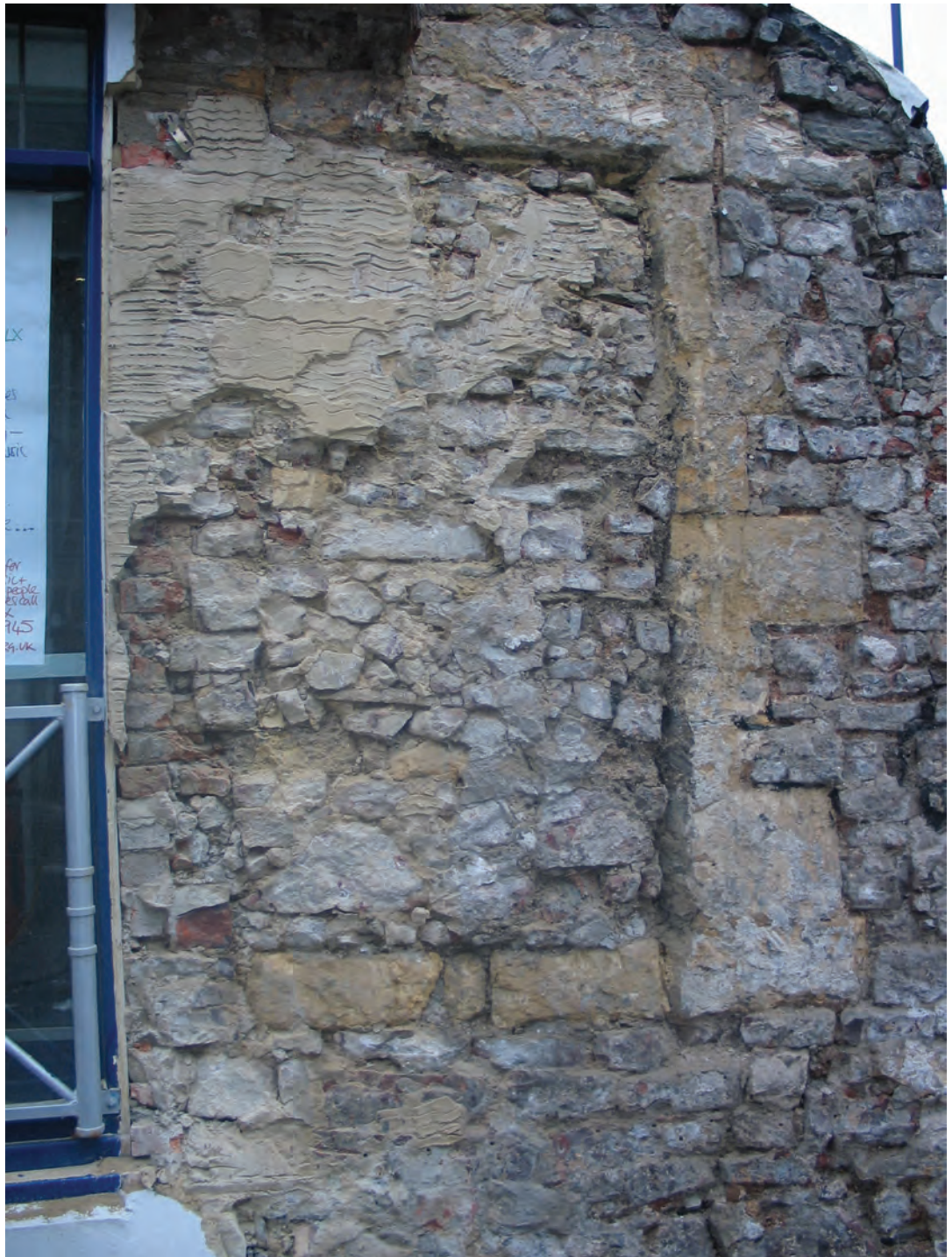
Figure 7.38 Remains of a possibly 16th-century window within No 2 Trenchard St (photograph R. Jones)
