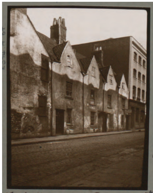
Figure 7.9 17th-century houses in Rosemary Street in 1931, demolished in 1954 (photograph by P E W Street, Bristol Museum and Art Gallery R394.A.87)
