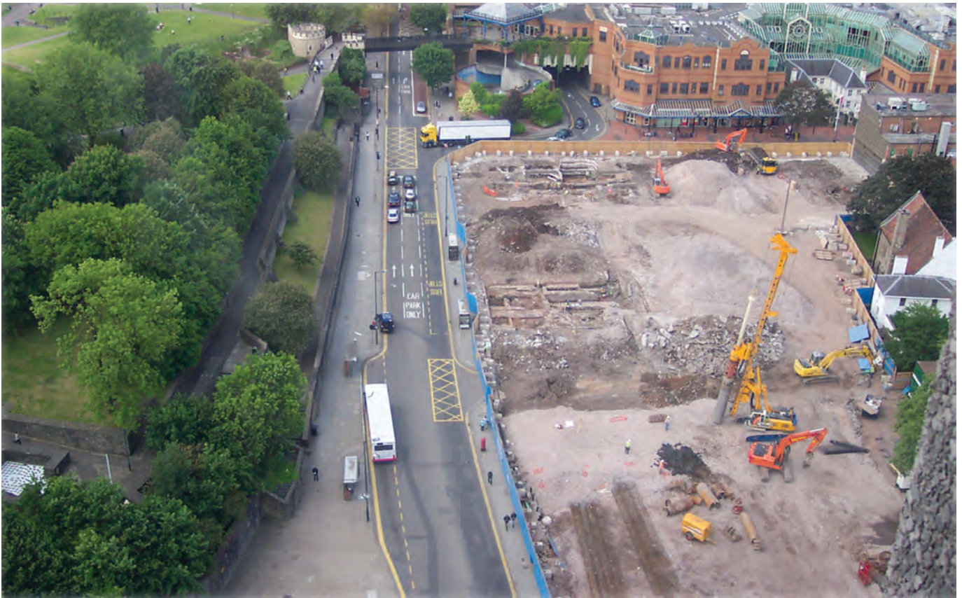
Figure 6.5 General view of Cabot Circus (Quakers Friars) excavation, 2005–6 (reproduced from Ridgenway and Watts 2013, fig 1.3)
