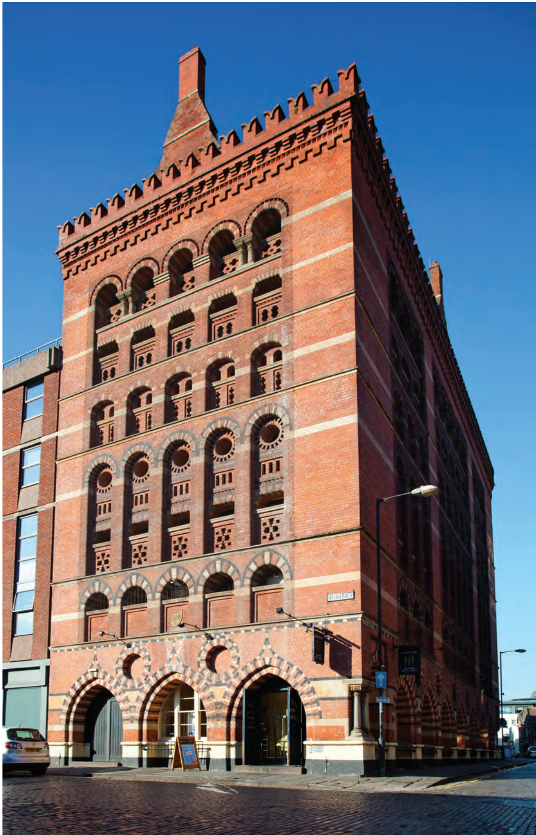
Figure 8.77 The Granary, Welsh Back (photograph D Martyn)
