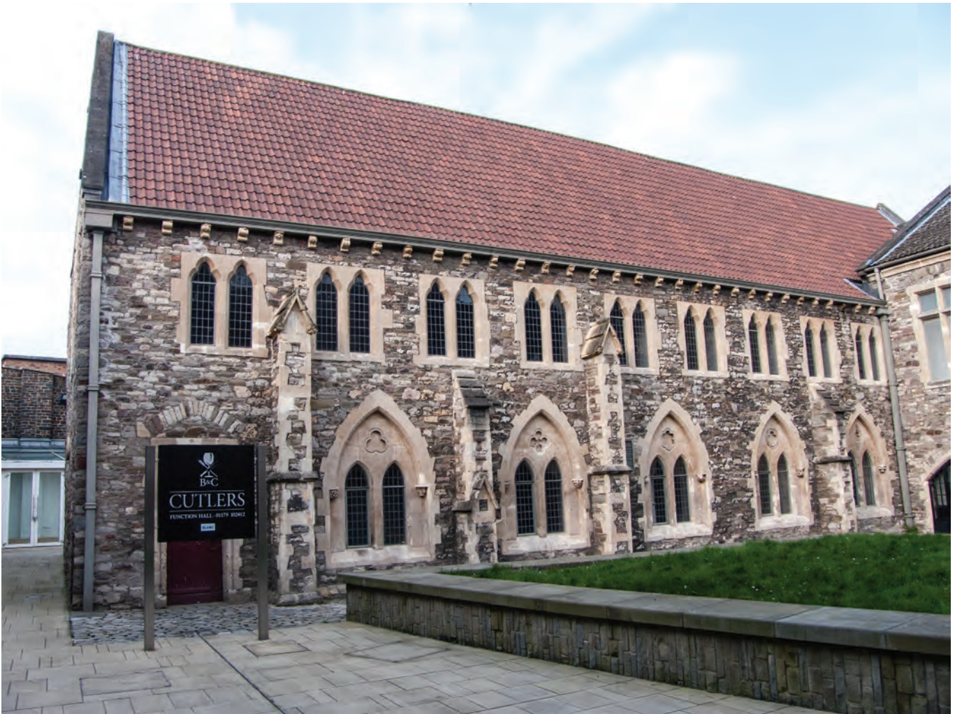
Figure 6.69 Cutlers Hall (photograph D Martyn)
