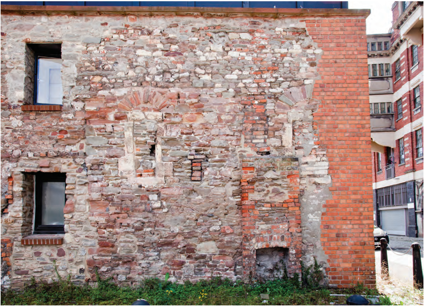
Figure 6.86 North wall of 'Canynge's Tower' in Redcliff Backs (photograph D Martyn)
