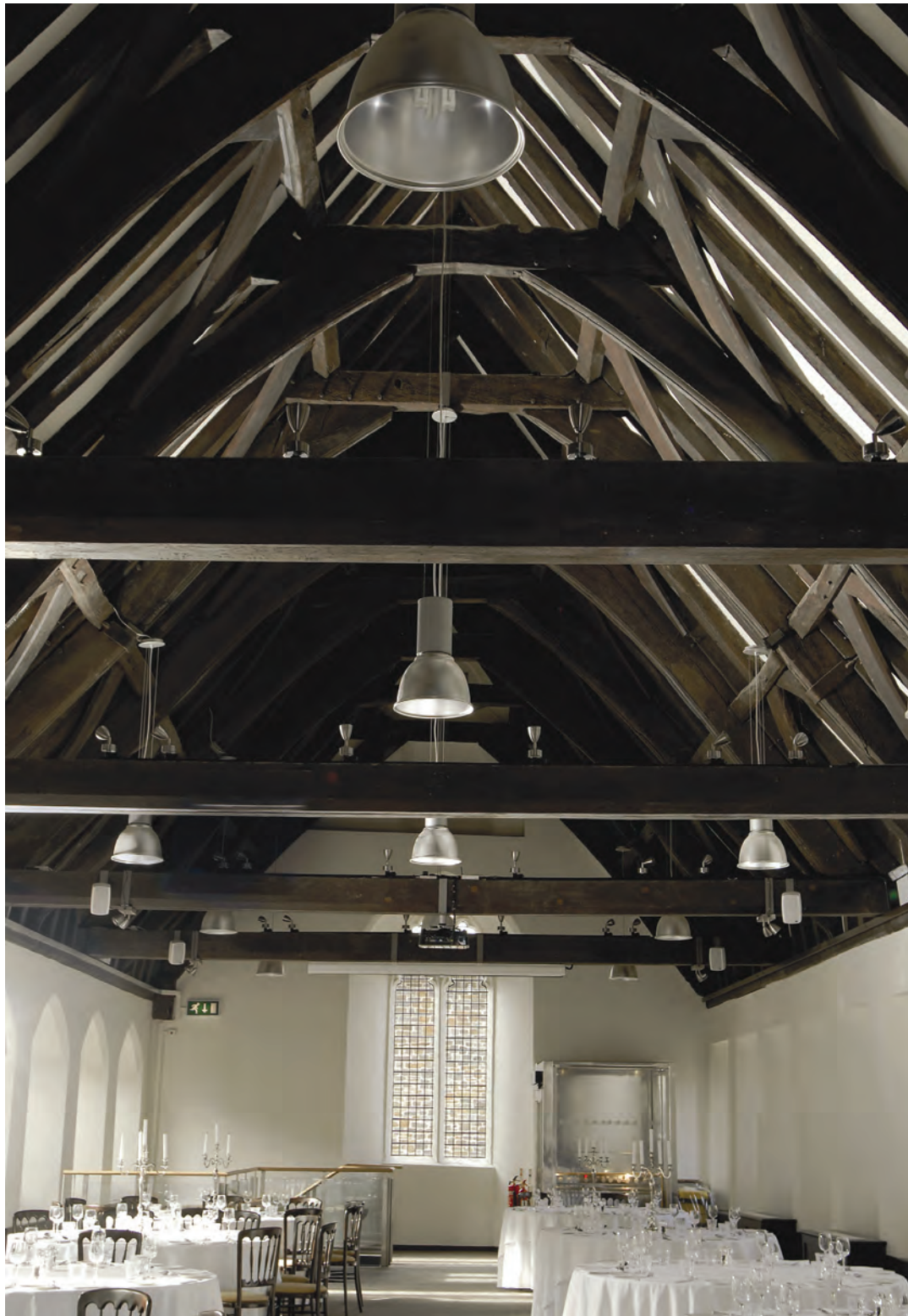
Figure 6.70 Roof of Cutlers Hall (photograph R. Jones)
