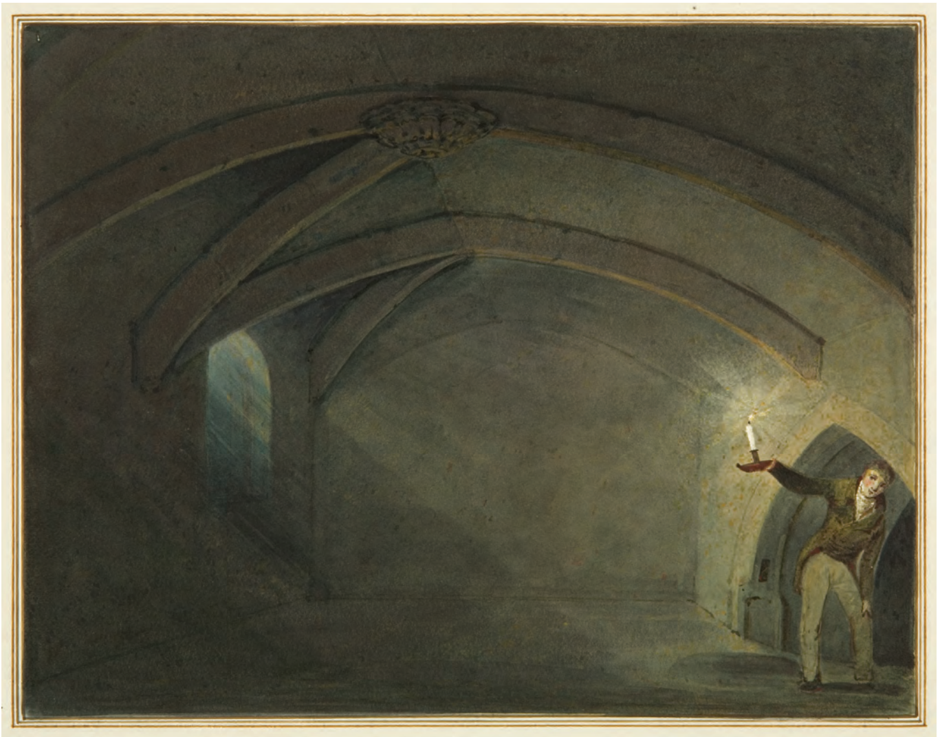
Figure 6.93 Vaults under No 32 Corn Street in 1827 by T L Rombotham (Braikenridge Collection, BRSMG M2294)
