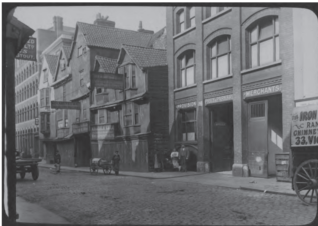
Figure 3.18 East side of St Thomas Street, 1906 (Bristol Archives, Bristol Municipal Charities Collection, ref 33041/BMC/12/1/b/46)
