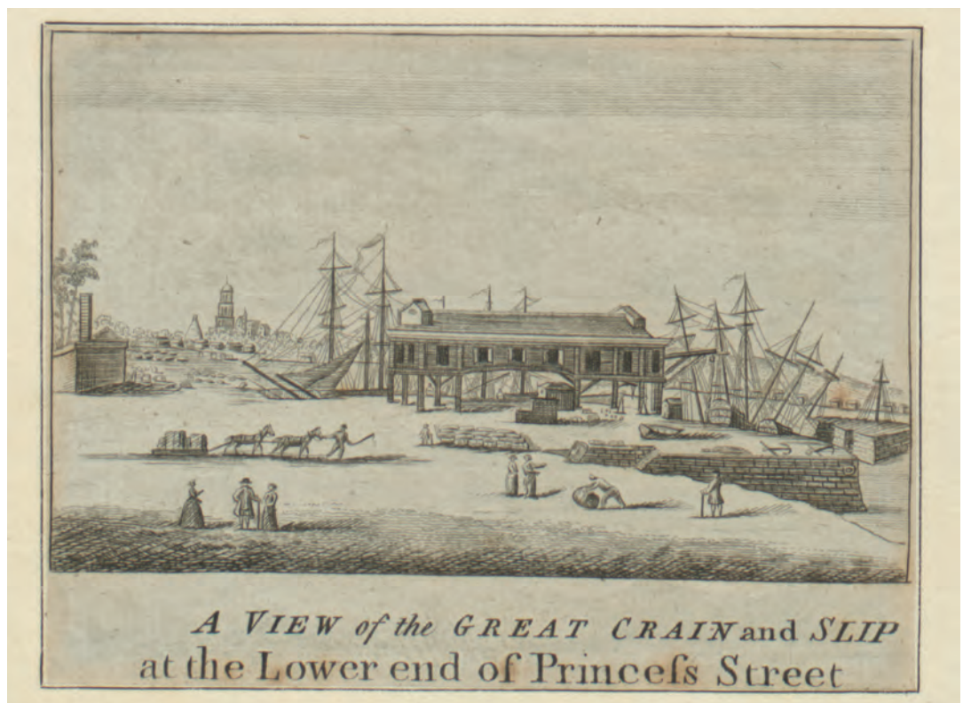
Figure 8.42 The Great Crane, erected 1735 (Bristol Reference Library collections. Braik.IV.159)
