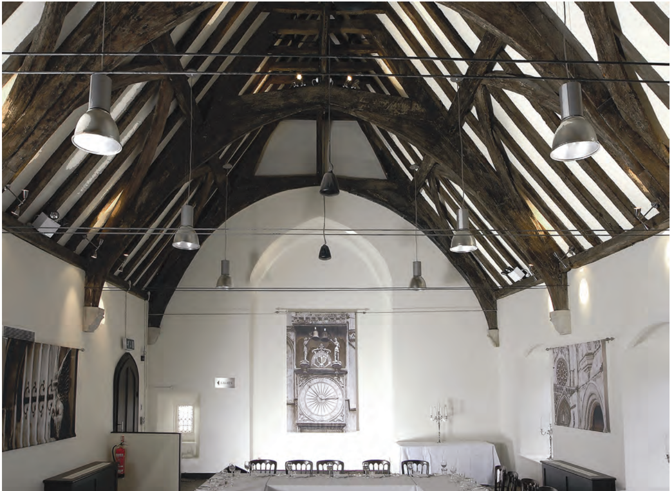
Figure 6.72 Roof of Bakers Hall (photograph R Jones)
