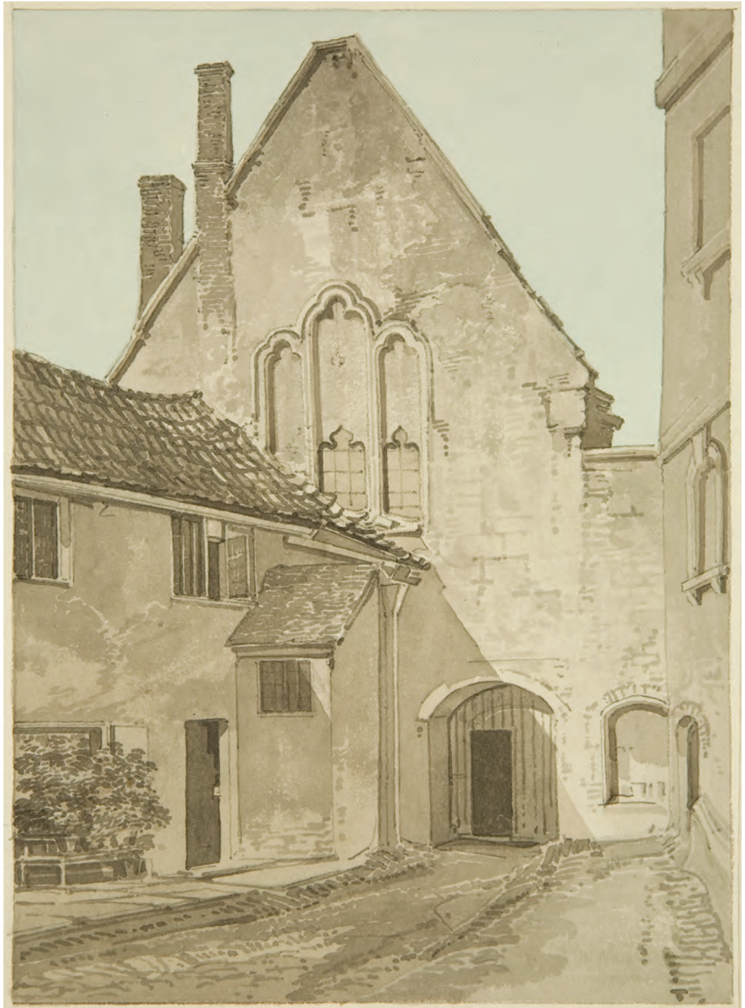
Figure 8.99 East window of Bakers Hall in 1821, before removal to Cutlers Hall, by Hugh O'Neill (Braikenridge Collection, BRSMG M2860)
