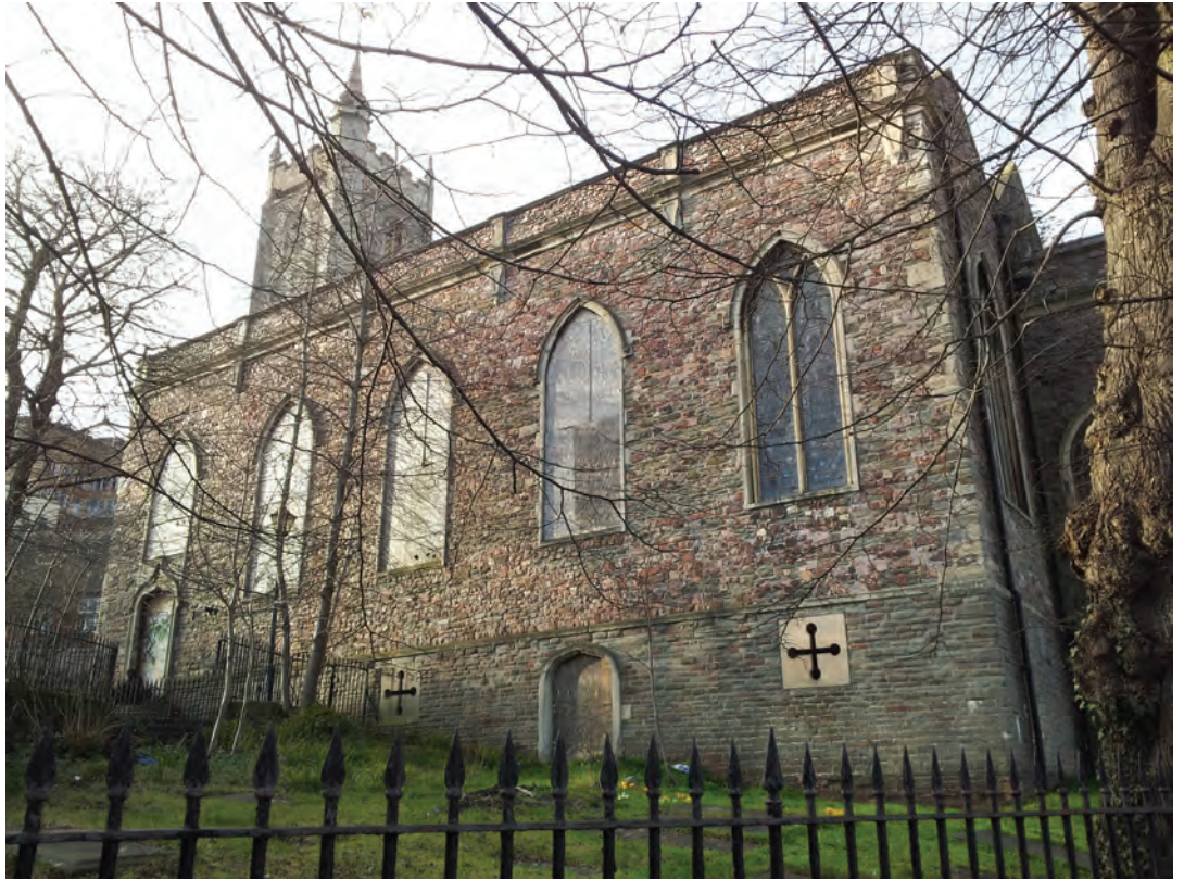
Figure 8.26 St Michael-on-the-Mount Church from the south-west (photograph D Martyn)
