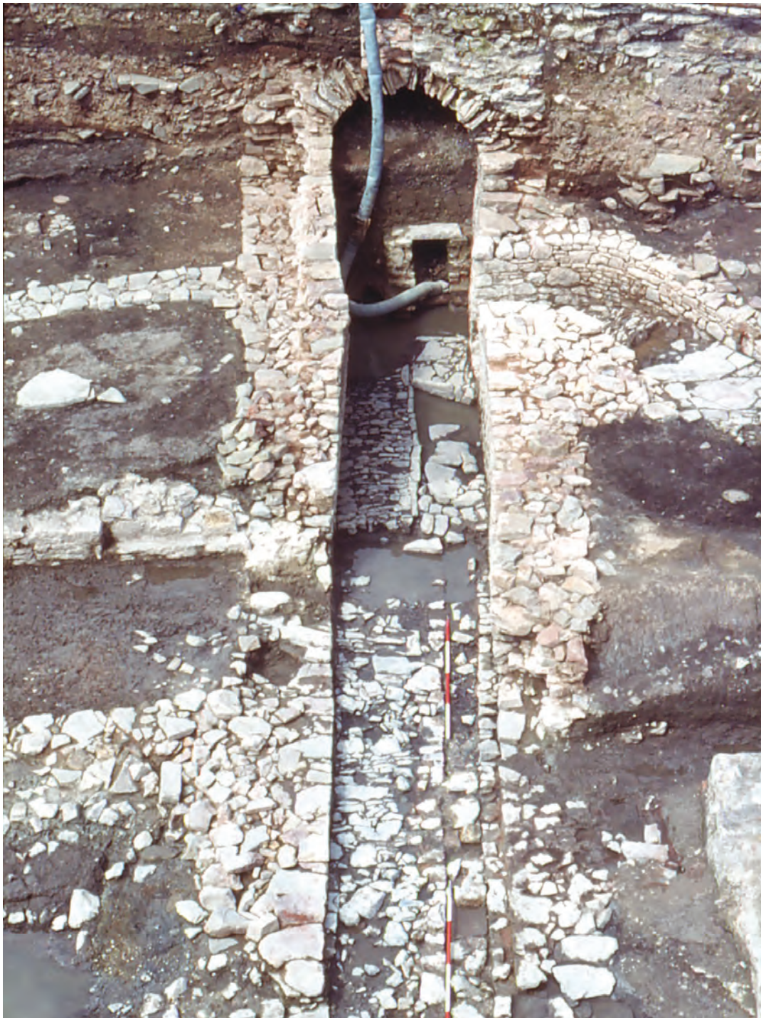
Figure 6.18 Nos 127–9 Redcliff Street. Medieval slipway looking towards the river
