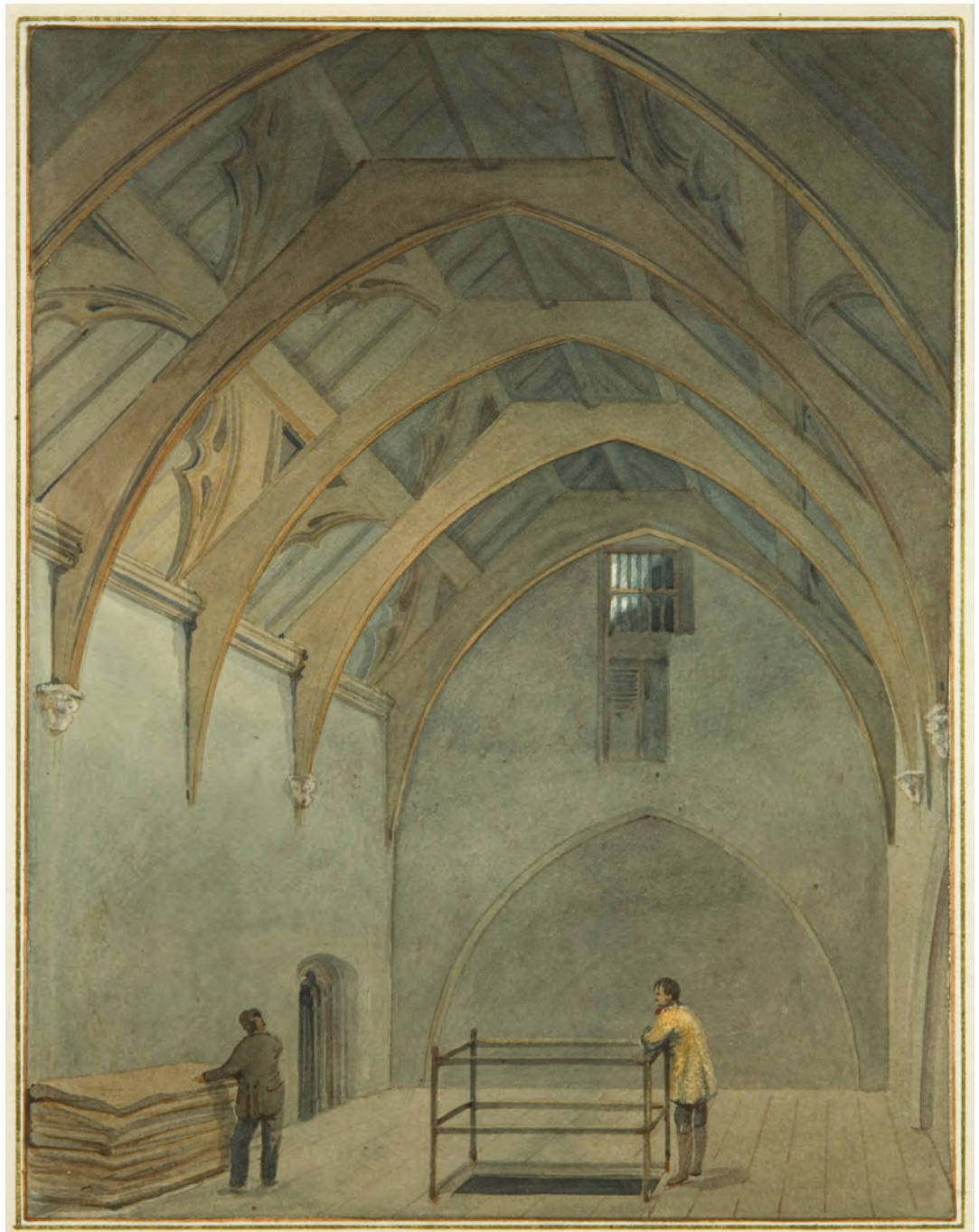
Figure 6.81 Spicer's Hall, looking north in 1826. Note the inserted first floor, with arches in the north and west walls extending below and the top of a window in the east wall, by T L Rowbotham (Braikenridge Collection, BRSMG M2244)
