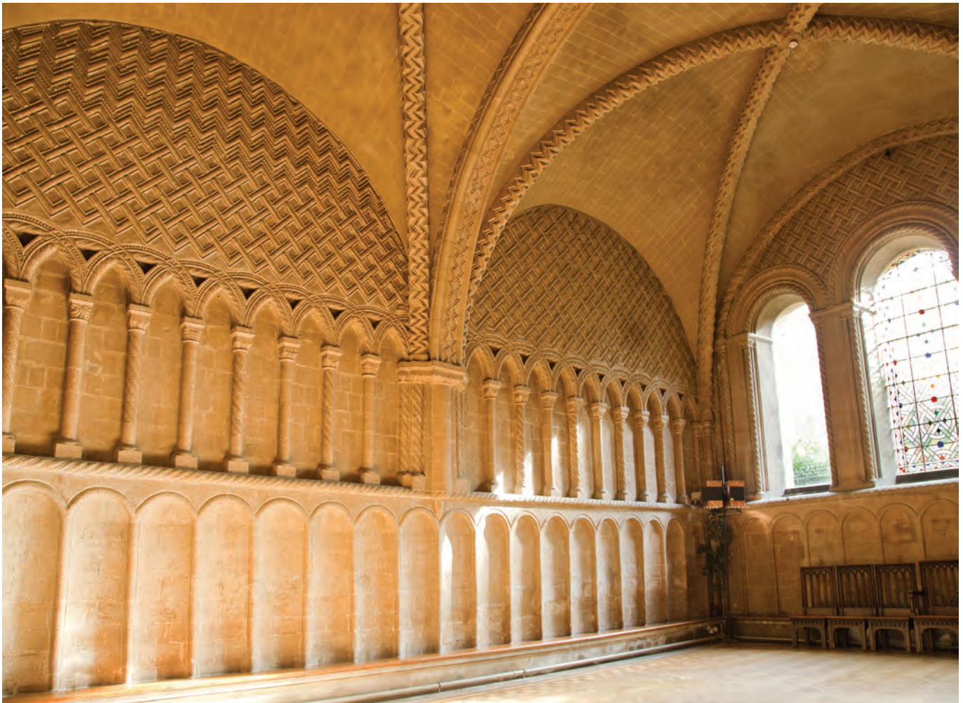
Figure 5.24 Lunettes above the blind arcade in the Chapter House (photograph D Martyn)
