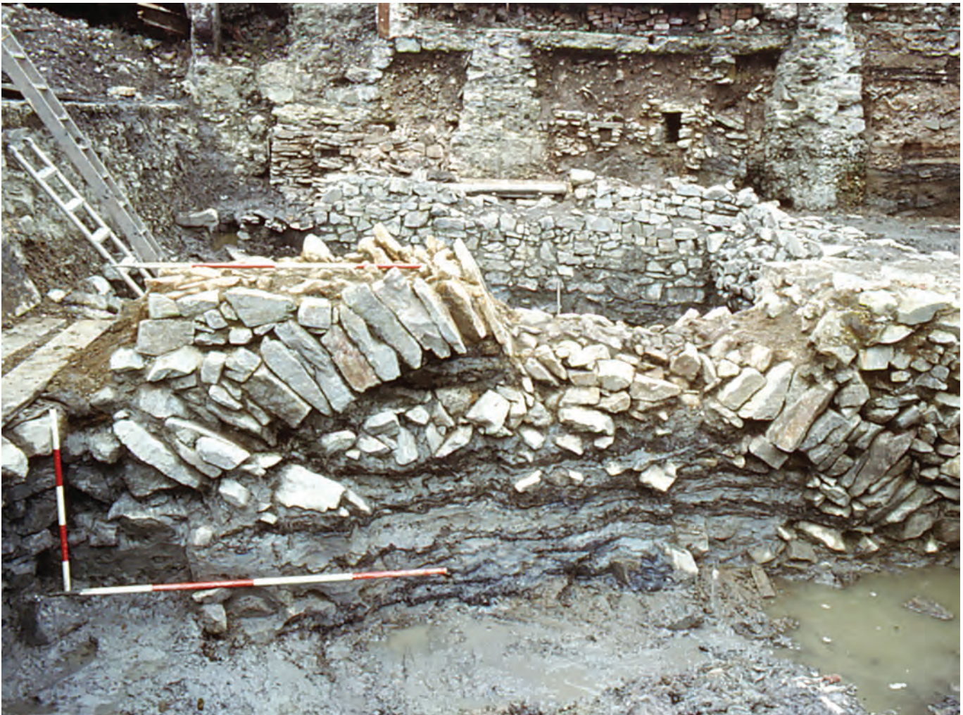
Figure 6.15 Stone waterfront revetment wall at Nos 127–9 Redcliff Street
