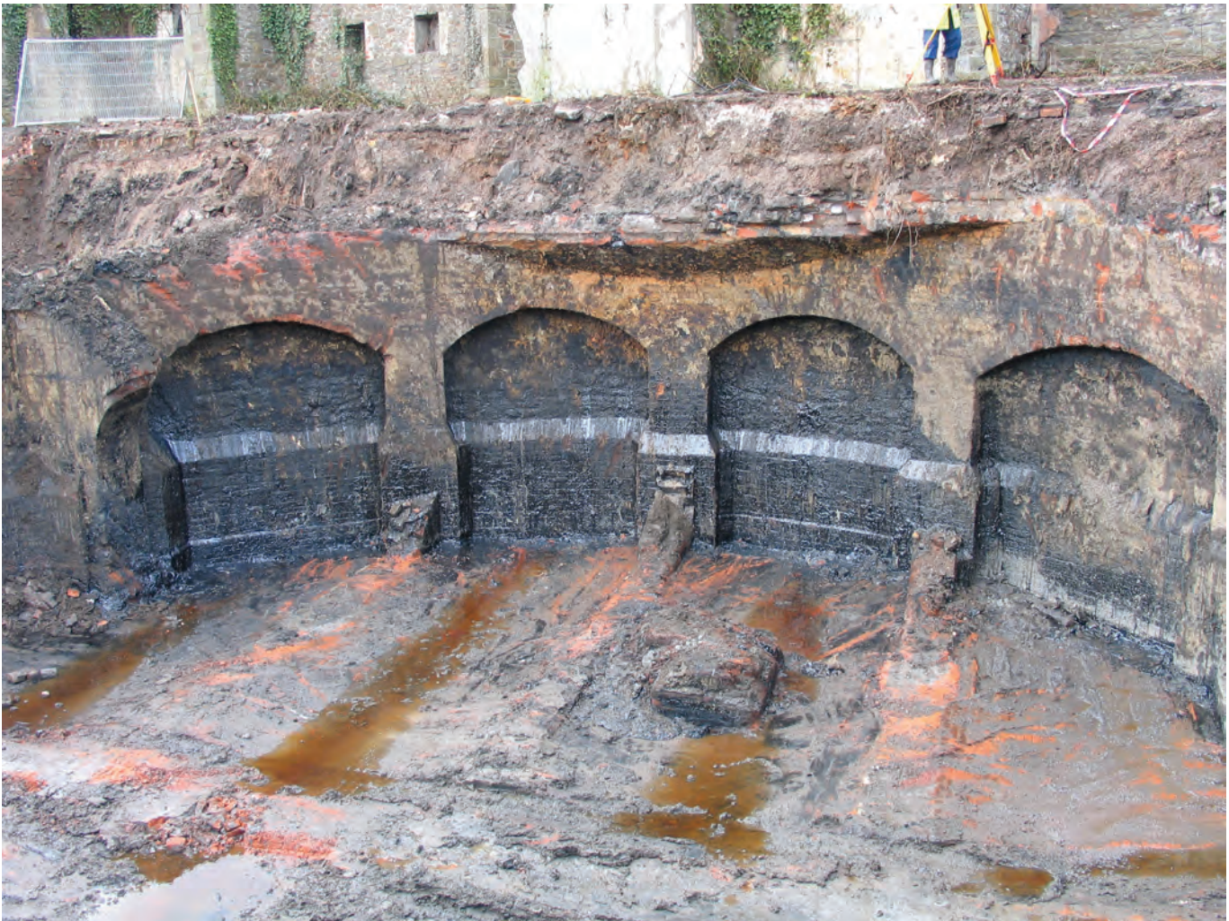
Figure 8.66 1840s gasholder, Canon's Marsh gasworks, during remediation and investigation in 2003 (photograph R. Jones)
