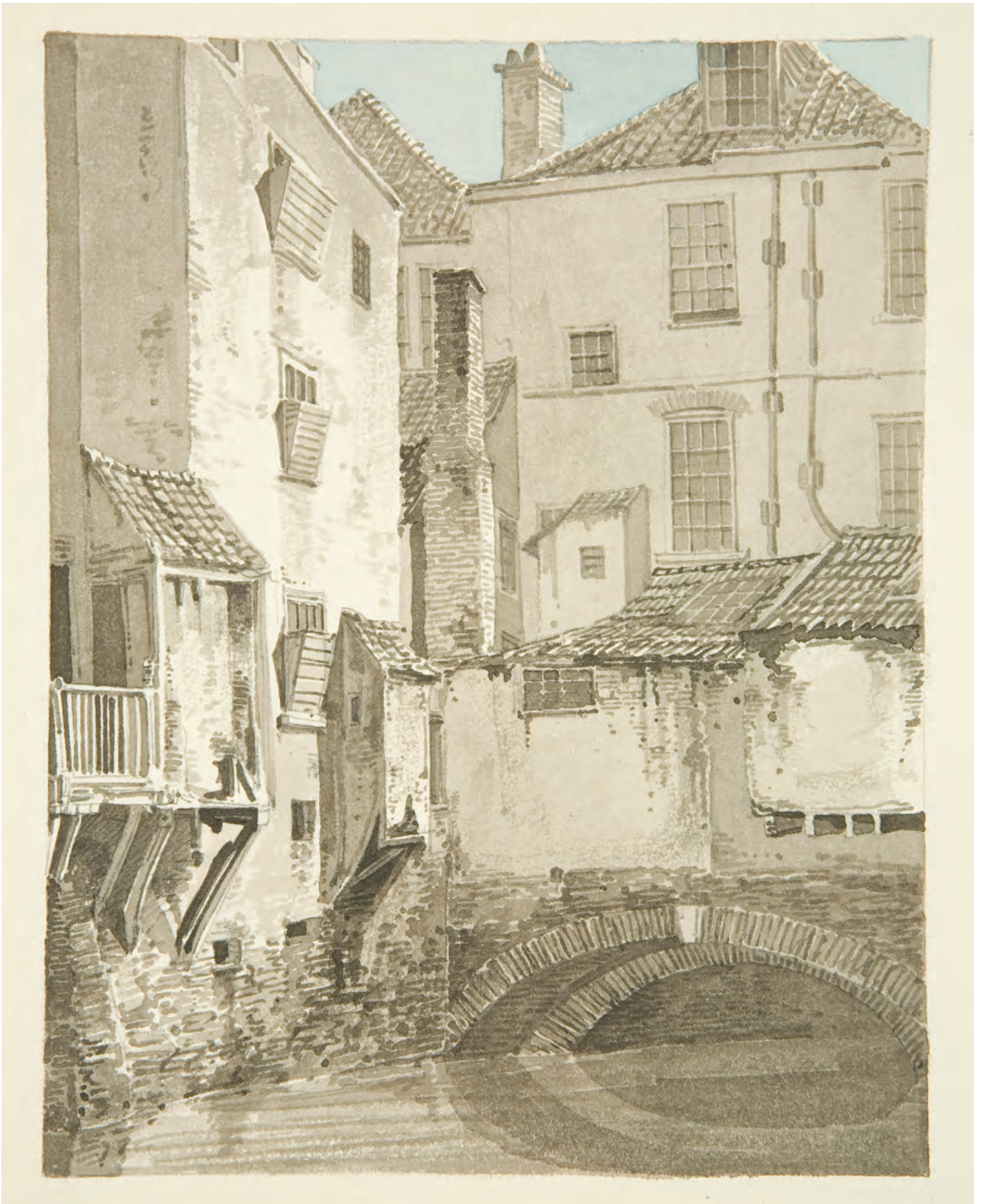
Figure 8.16 Rear of a building on St John's Bridge adjacent to Frome Bridge, showing overhanging privies in 1821 by Hugh O'Neill (Braikenridge Collection, BRSMG M2894)
