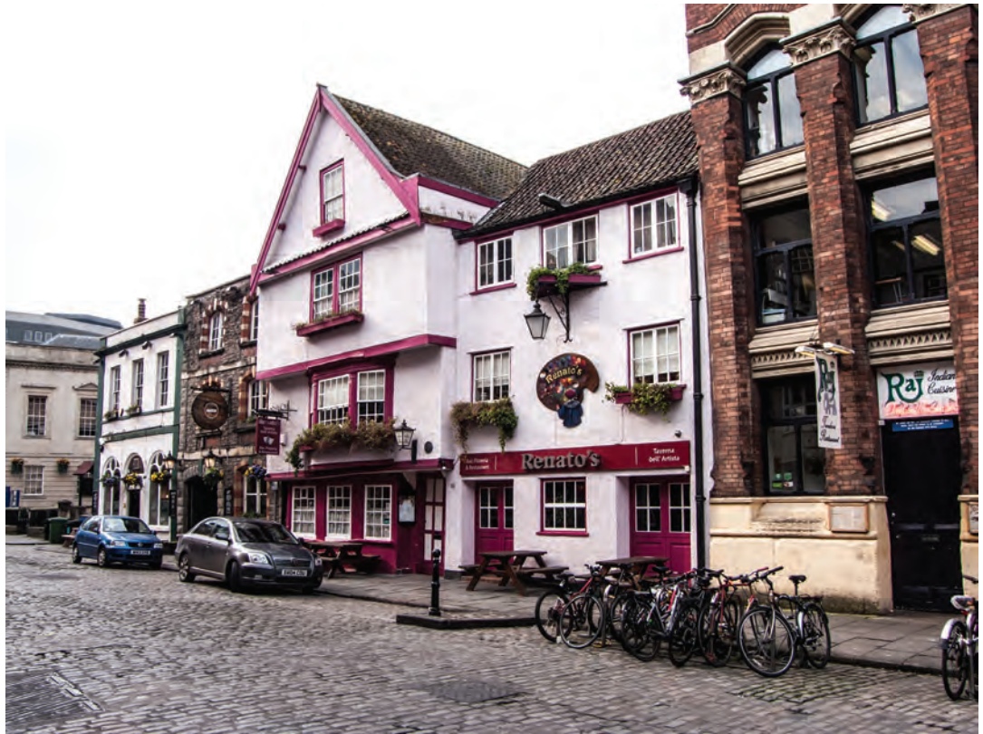
Figure 7.17 33 King Street (photograph R. Jones)
