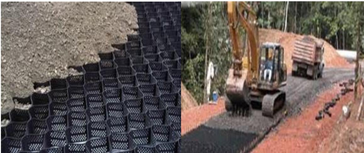
**Figura N° 5: Geoceldas**
