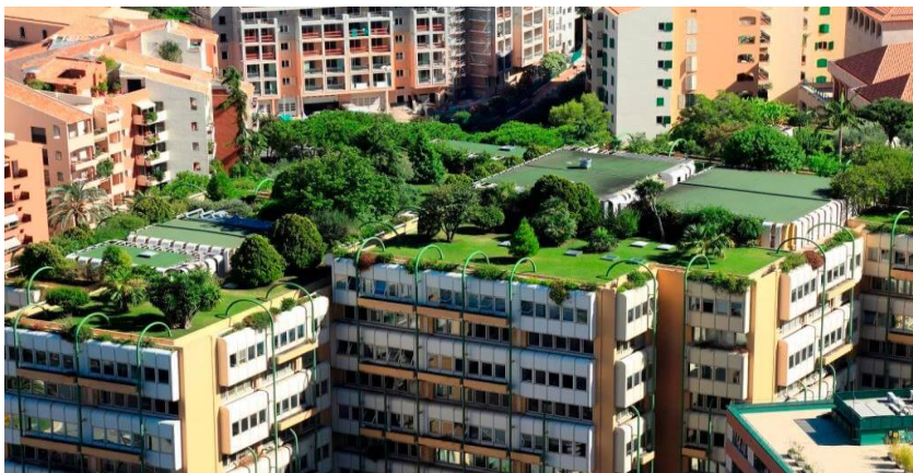
Figure 3. Green roofing technique [25].
