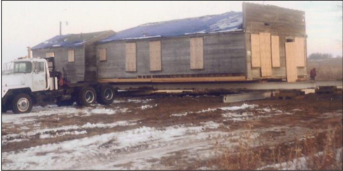
Figure 21. Moving the Jackson House temporarily off its original site in 2001. Photo courtesy of Kevin Murray, Bellvue, Colorado.
