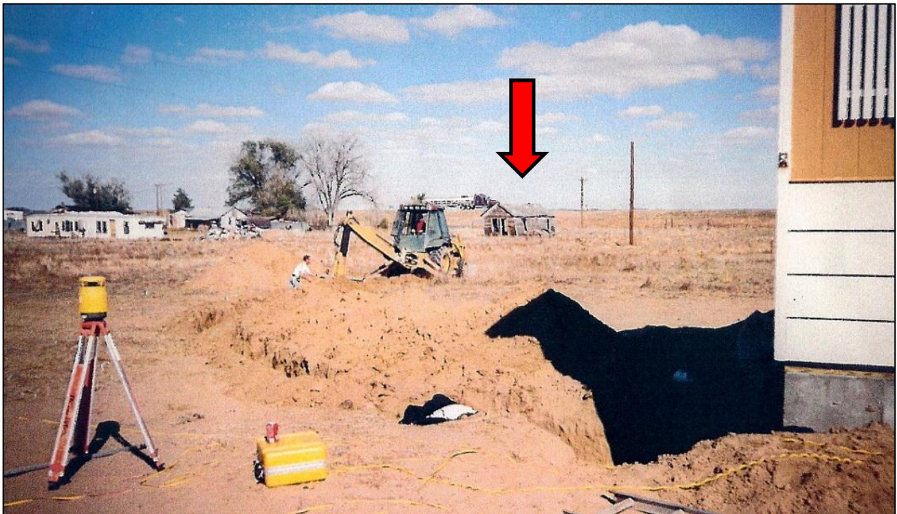
Figure 6. 2003 photo of block 4 house from adjacent neighbor's house.
