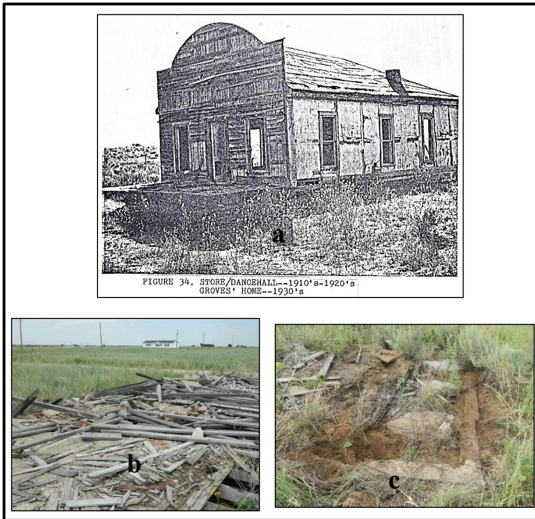
Figure 33. a) photograph from Norris 1980: Figure 34 of the Store/Dance Pavilion while still standing in the 1970s; b) overview of the collapsed store in 2011; c) photo of the small outlying structure (with well-defined concrete foundation) suspected being privy.
