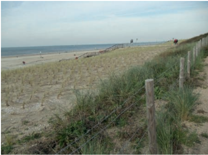
Figure 9.3 Widening and extending the dune ridges seaward and replanting with native vegetation along the Delfland coast, The Netherlands, 2013.
