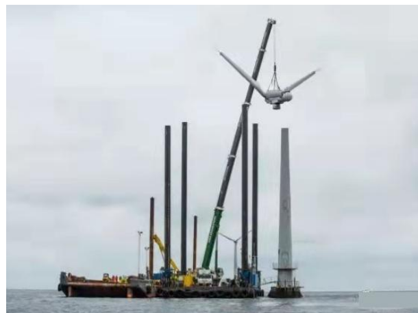
Figure 2.3 The decommissioning of the world's first OWF - Vindeby
