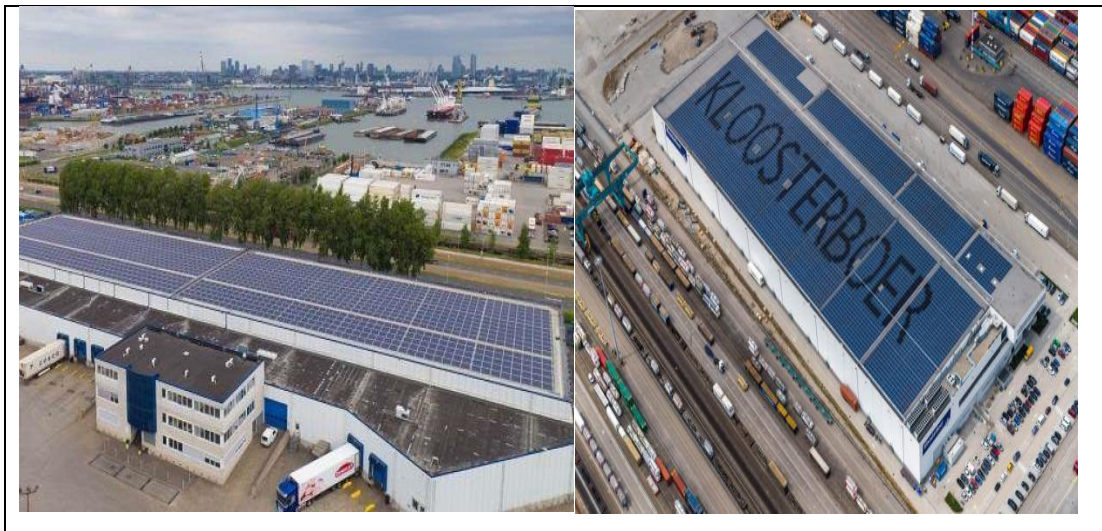
Figure 8: Solar panels on the rooftop of the warehouse at Port of Rotterdam (Marasi News, 2016).
