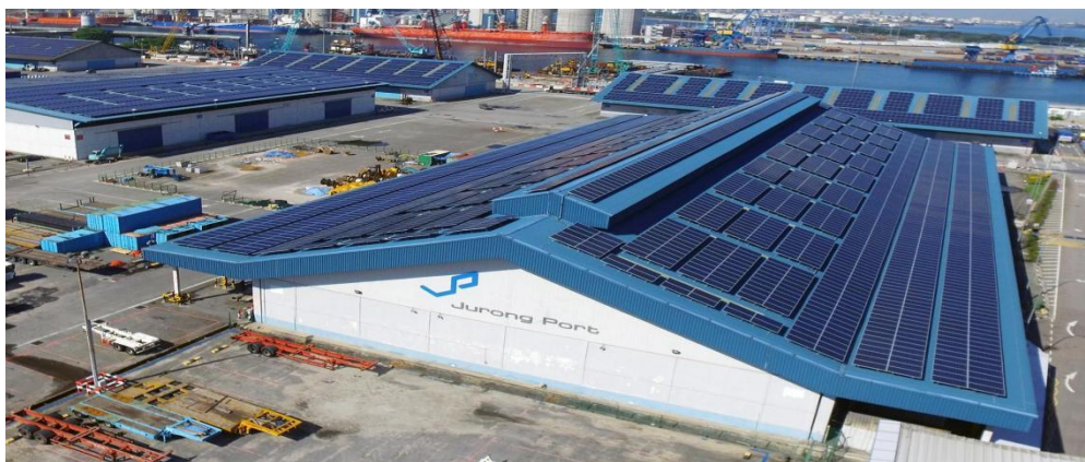
Figure 9: Solar panels at Jurong port (Bantillo, 2016).
