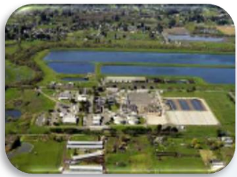
Waste Water Treatment Plant
