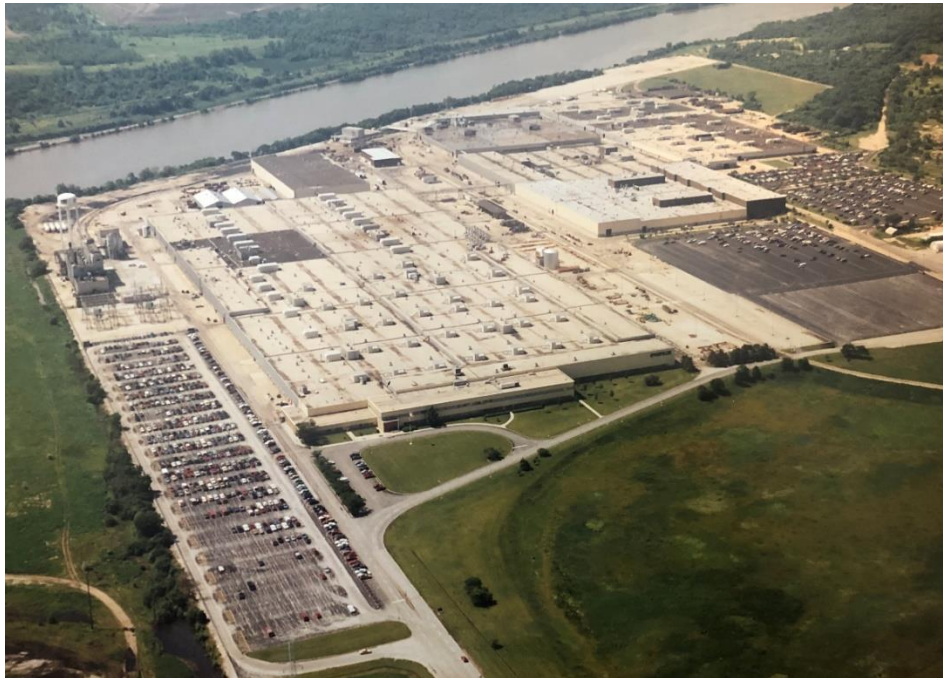
Figure 2. Historical photograph of the Caterpillar Joliet plant, May 1991. Public domain.
