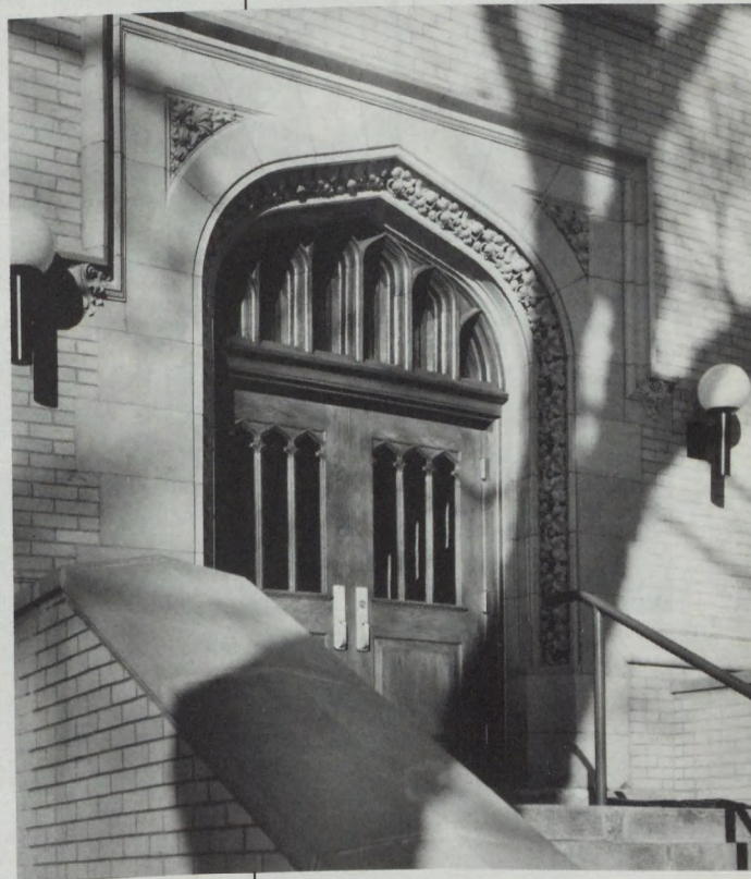
As with the Scovel renovation, Bogner Construction Co. preserved the best of the old in its work on Taylor.
