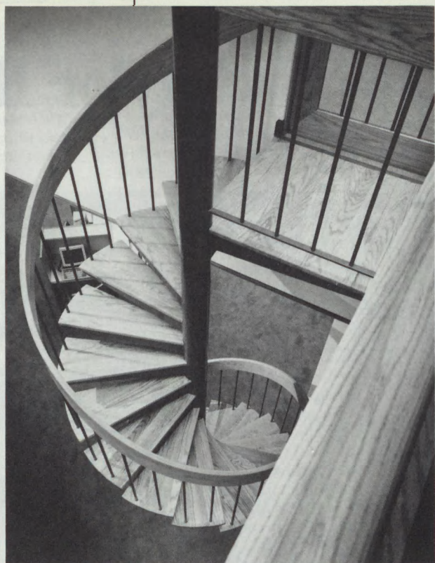
The atrium's circular staircase, descending into what was once the second floor lounge.
