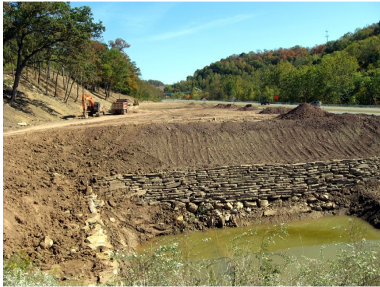
Figure 11. Change in hydrologic regime within study area. The area was filled following the survey period, eliminating a wetland and altering the drainage pattern.
