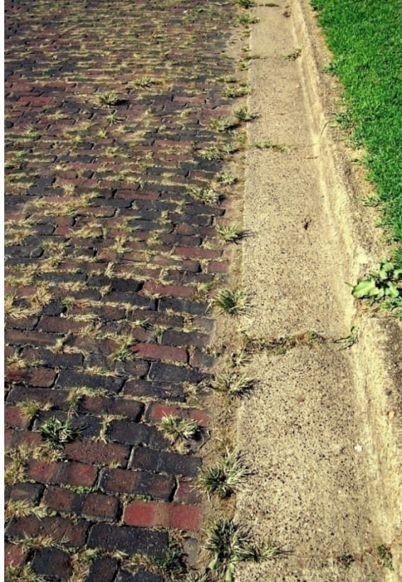
Figure 23. Gradient of interstitial vegetation decreasing from edge to center of roadway.
