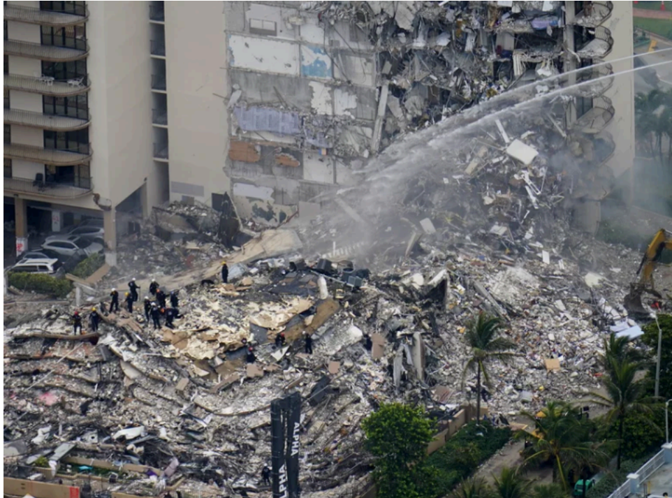
Figure 11 the collapsed South Chaplain Tower [20]
