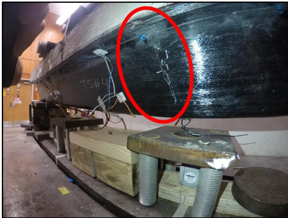
Figure 37: Web Failure of Specimen 4
