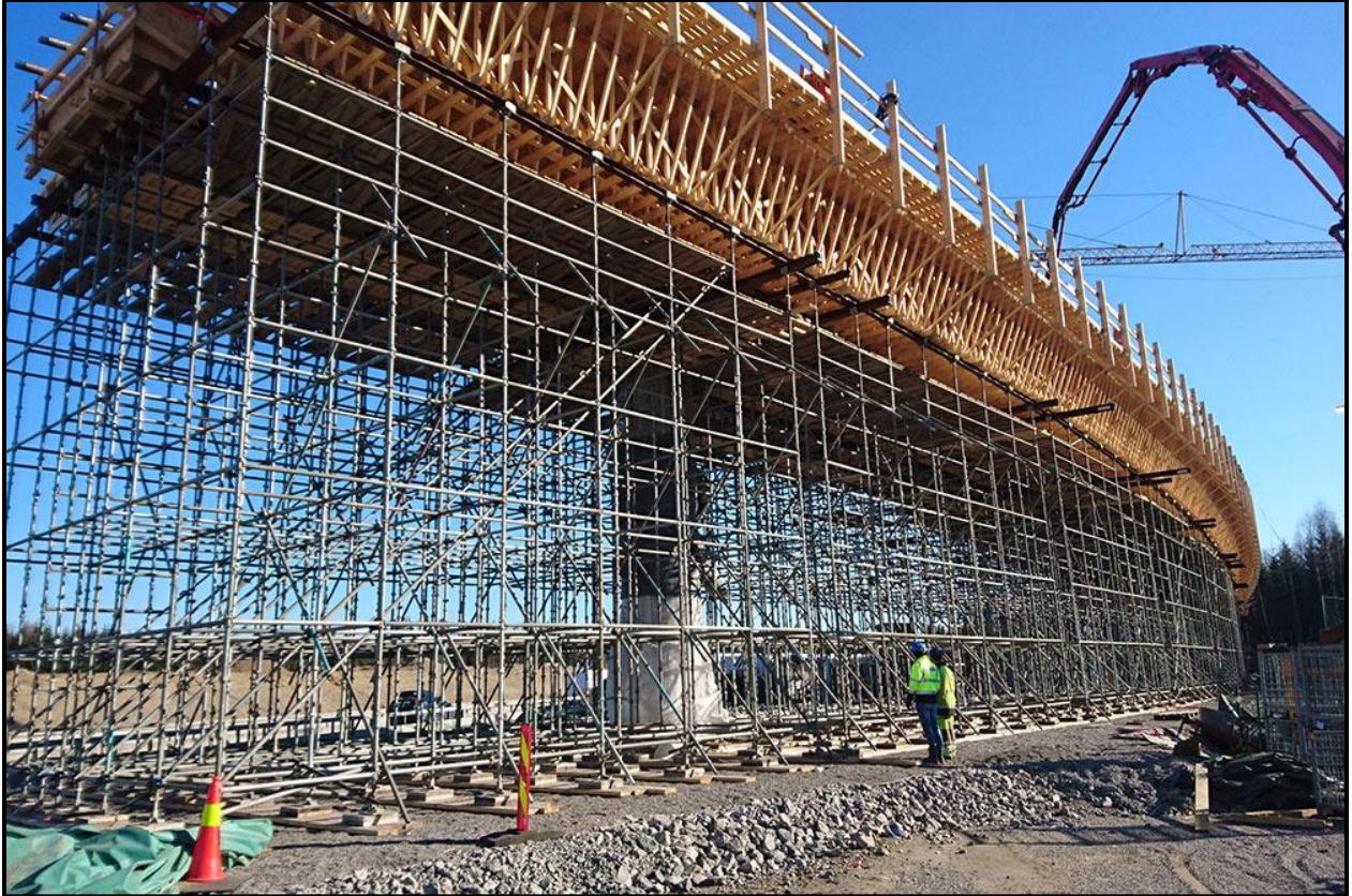
Figure 1: Temporary Formwork for Concrete during Bridge Construction [1]
