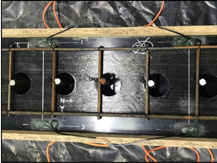
Figure 26: Rebar Cage and Formwork Prepared for Concrete
