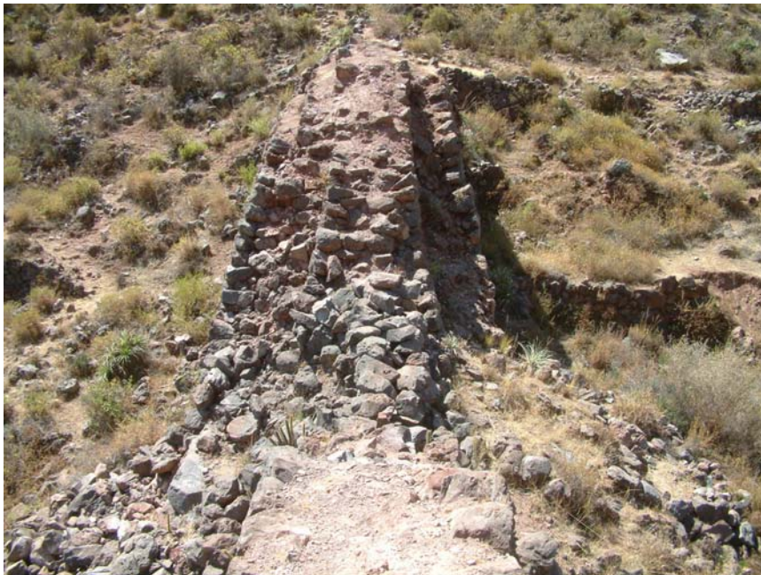
Figure 15. The Combayoc aqueduct is less well known than the Rumicolca aqueduct, yet it is also impressive.
