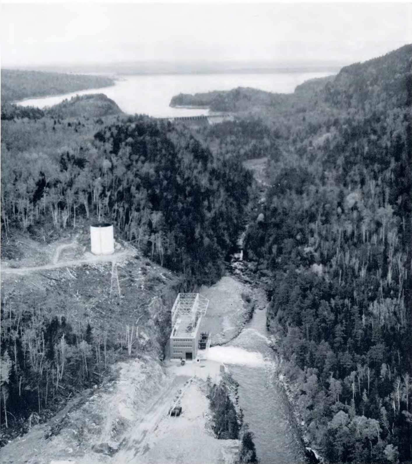
Ripogenus Dam and McKay Station. This dam impounds 30 billion cubic feet of water in Ripogenus and Chesuncook Lakes. The power station takes water from the dam through a 4,100-foot pressure tunnel.
