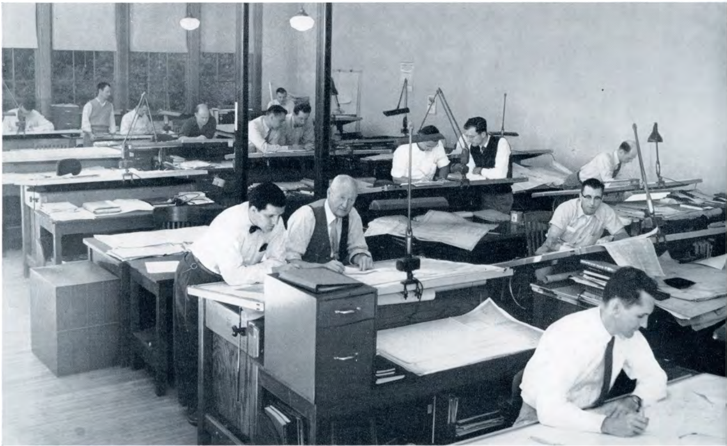
Practically every phase of engineering is involved in the operation and maintenance of a newsprint mill. A large portion of the design for the new construction at East Millinocket is being handled by Great Northern's own engineering organization. This picture shows part of the engineering staff at work.
