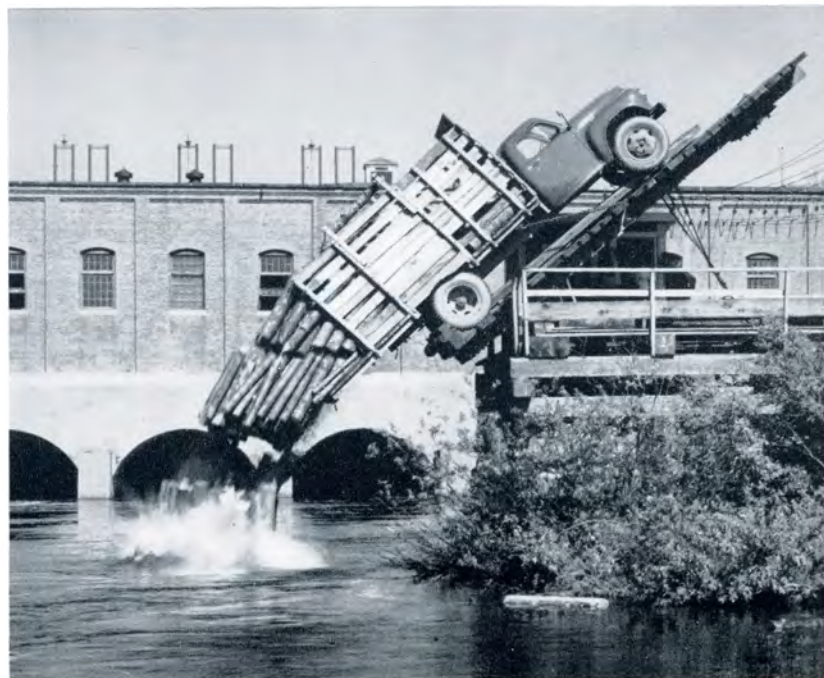
(Below) Unloading truck wood in the easy way. The truck is backed on to the platform, is chained down, and five cords of wood are dumped in no time.
