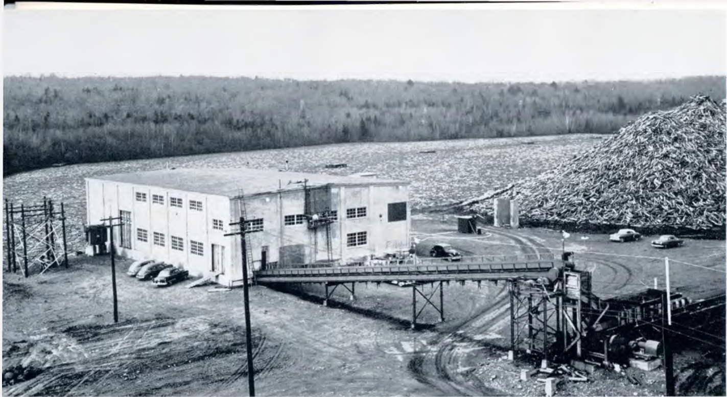
New wood room at East Millinocket Mill, the first building to be put into use in the current expansion program. This building houses the drum barkers and hydraulic barking equipment.
