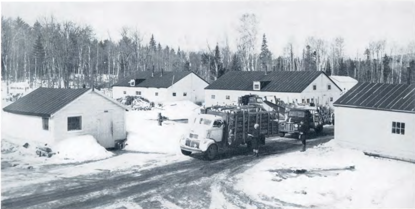
Modern camps for woodsmen are a far cry from the log buildings of 20 years ago. Here is a typical Great Northern camp today. The buildings are portable, and are equipped with electric lights, shower baths, refrigerators. Left to right: scaler's camp, cook shack, bunk house, repair shed and office.
