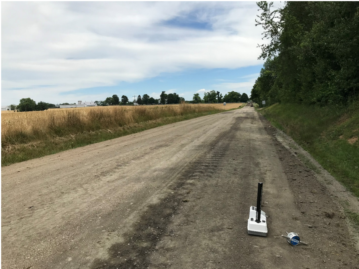
Figure 4.22 Shelby Co. CID 192383, KY 1779, Full Depth Reclamation of Existing Pavement Structure
