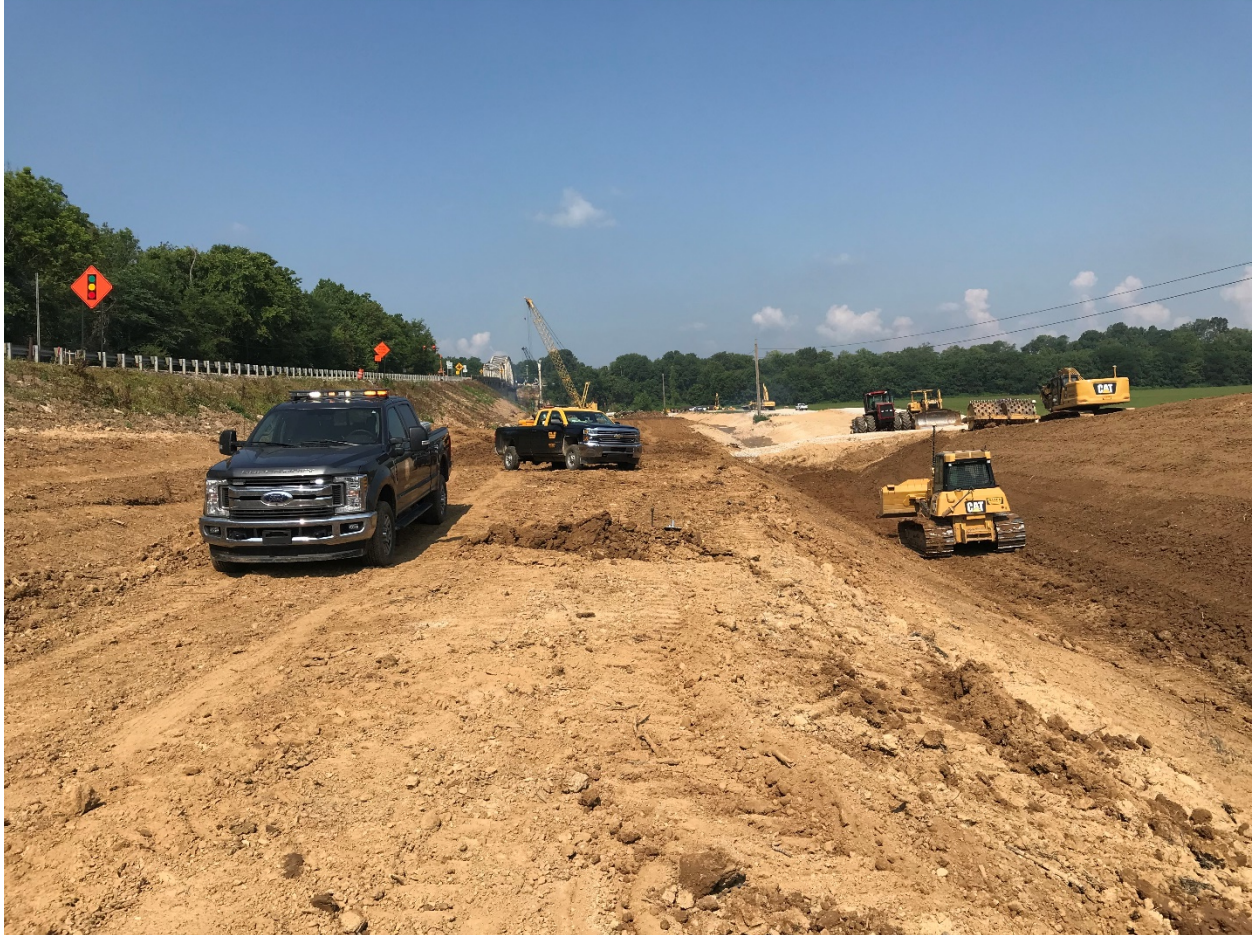
Figure 4.30 Henderson Co. CID 191247, US 60, New bridge over Green River at Spottsville
