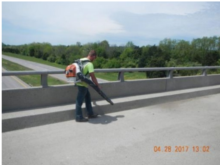
Figure 39 Cleaning gutter line of debris with a blower
