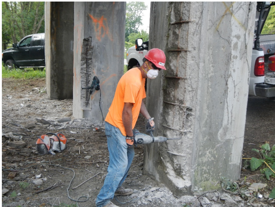
Figure 45 Mechanical removal of distressed concrete on a pier column
