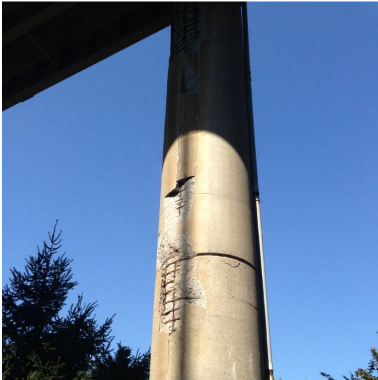
Figure 6 Concrete spalling on pier column with corroded reinforcing steel on I-65 approach span
