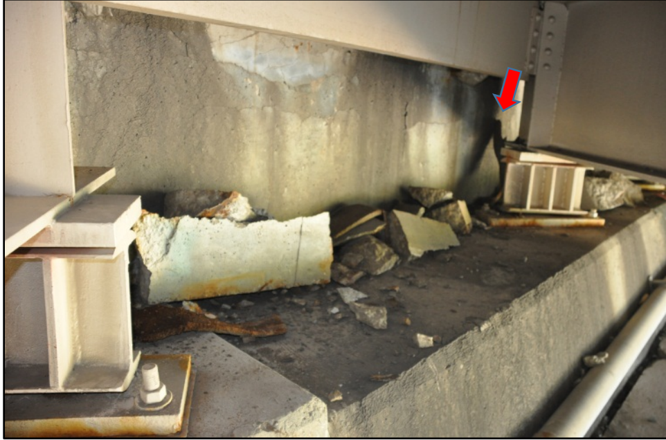
Figure 3 Deck joint failure with concrete spalling on the abutment backwall. note detached joint seal (arrow)
