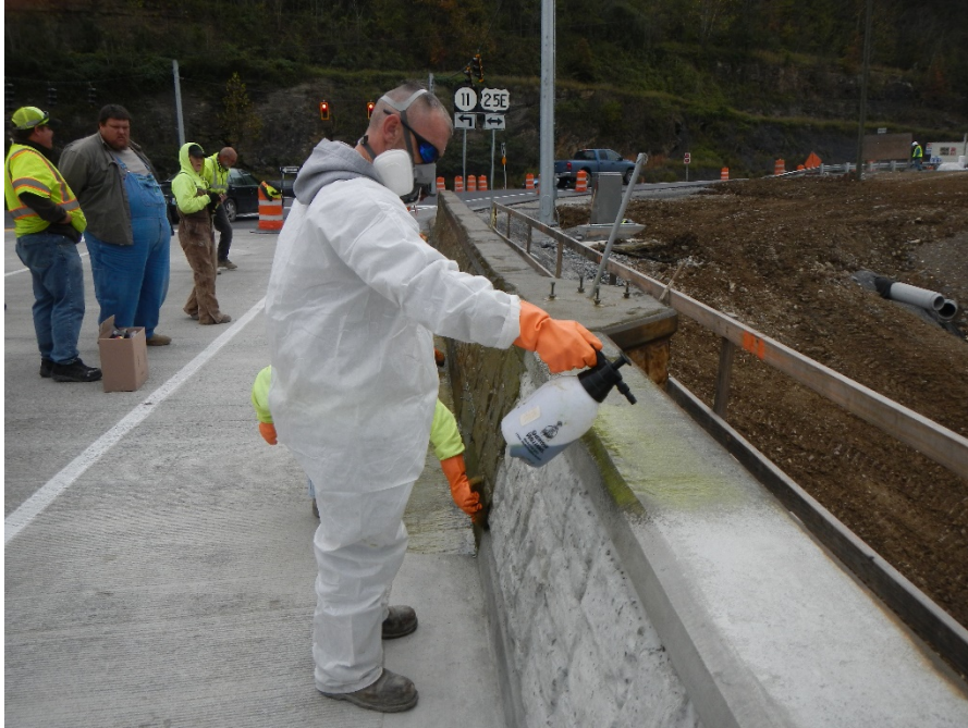
Figure 40 Hand sprayer application of a silane sealer on a barrier wall
