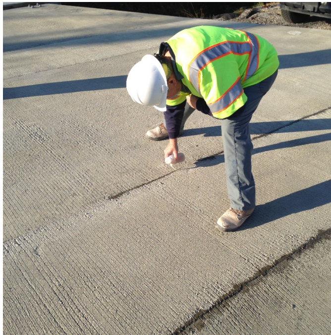
Figure 49 Sealing a cold joint in a bridge deck with methyl methacrylate
