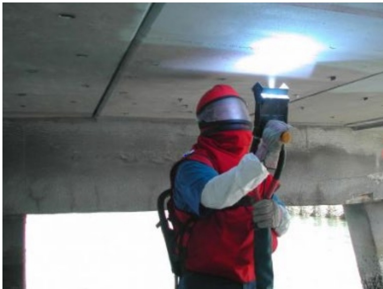
Figure 57 Sheet zinc galvanic anode being applied by metallizing concrete (courtesy Vector Corrosion Technologies)
