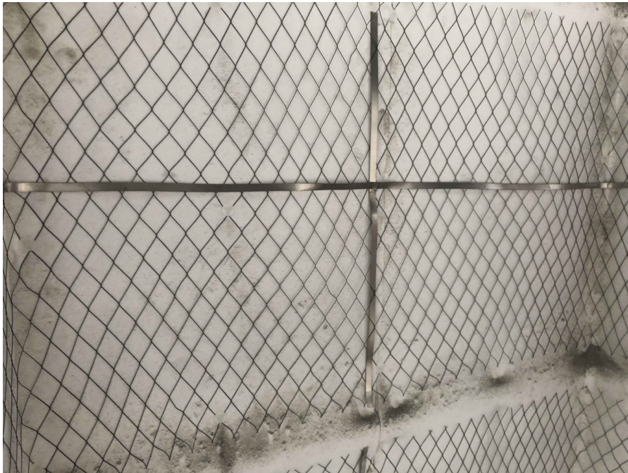
Figure 51 Metallic conductive mesh applied over conductive media for electrochemical extraction treatment (courtesy Vector Corrosion Technologies)
