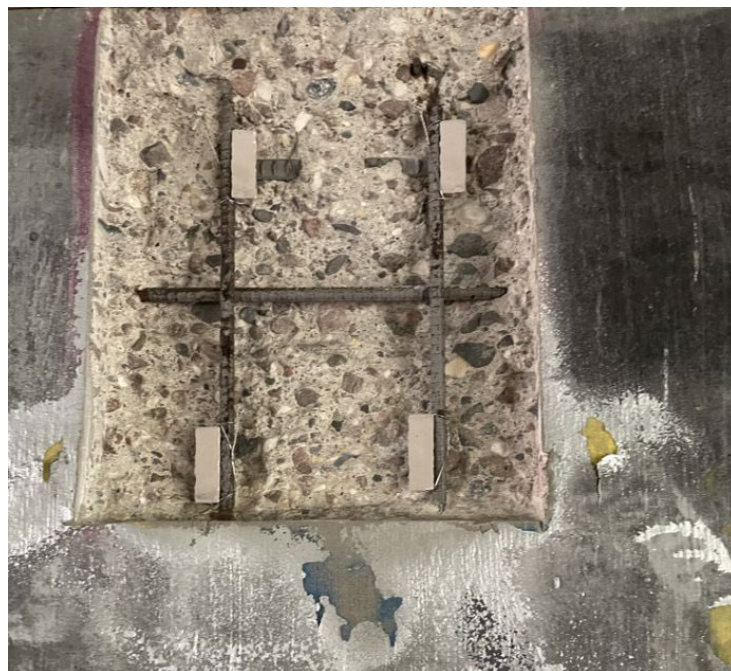
Figure 55 Four discrete galvanic anodes used in a patch repair (courtesy Vector Corrosion Technologies)
