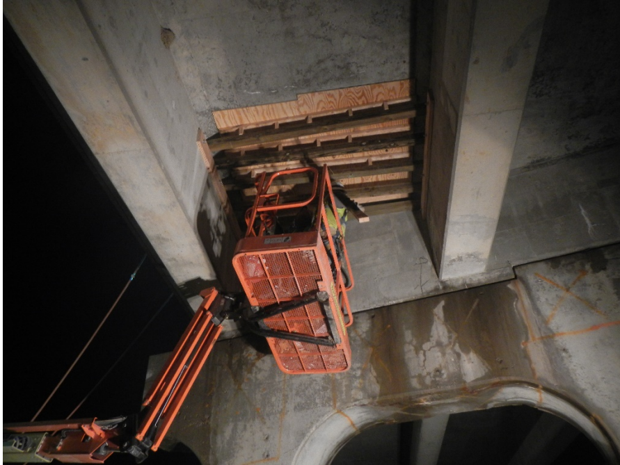
Figure 46 Formwork being installed on a deck overlay repair to accommodate a full depth patch
