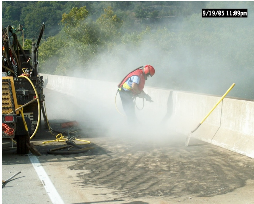
Figure 42 Abrasive blasting of a barrier wall prior to painting
