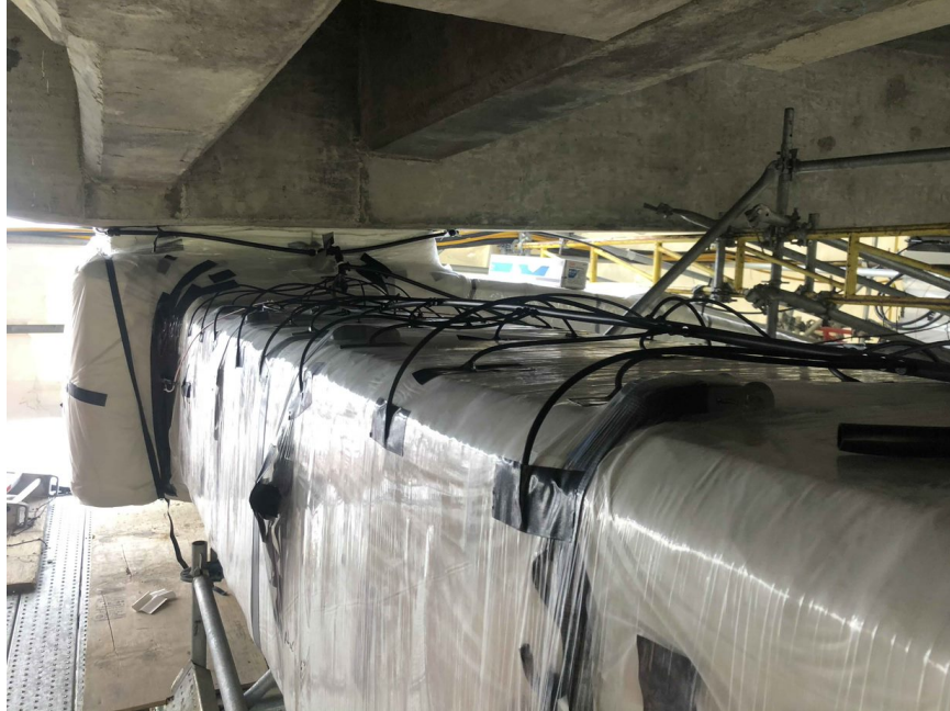
Figure 52 Wrapped girder undergoing electrochemical extraction treatment (courtesy Vector Corrosion Technologies)
