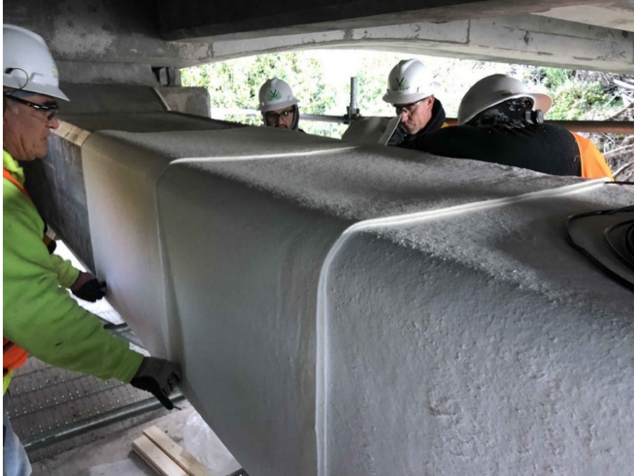
Figure 50 Applying conductive media wrap for electrochemical chloride extraction treatment (courtesy Vector Corrosion Technologies)
