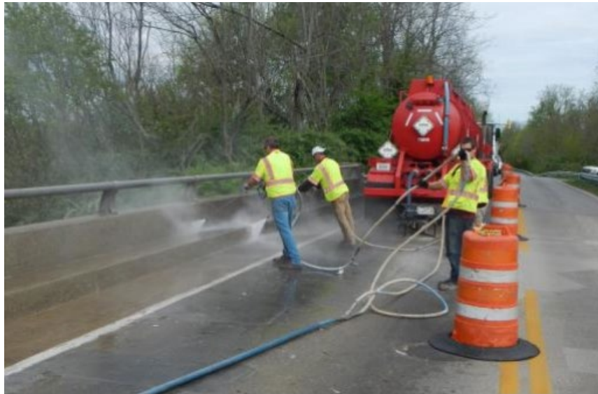
Figure 41 Pressure washing of a concrete barrier wall prior to painting
