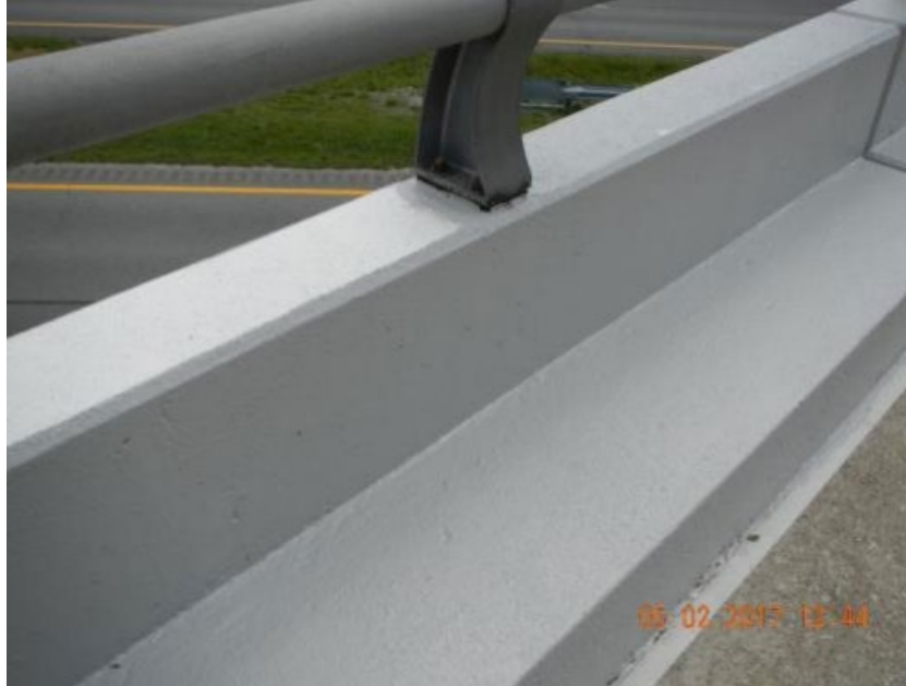
Figure 44 Painted concrete barrier wall with two-coat (epoxy-acrylic) paint system
