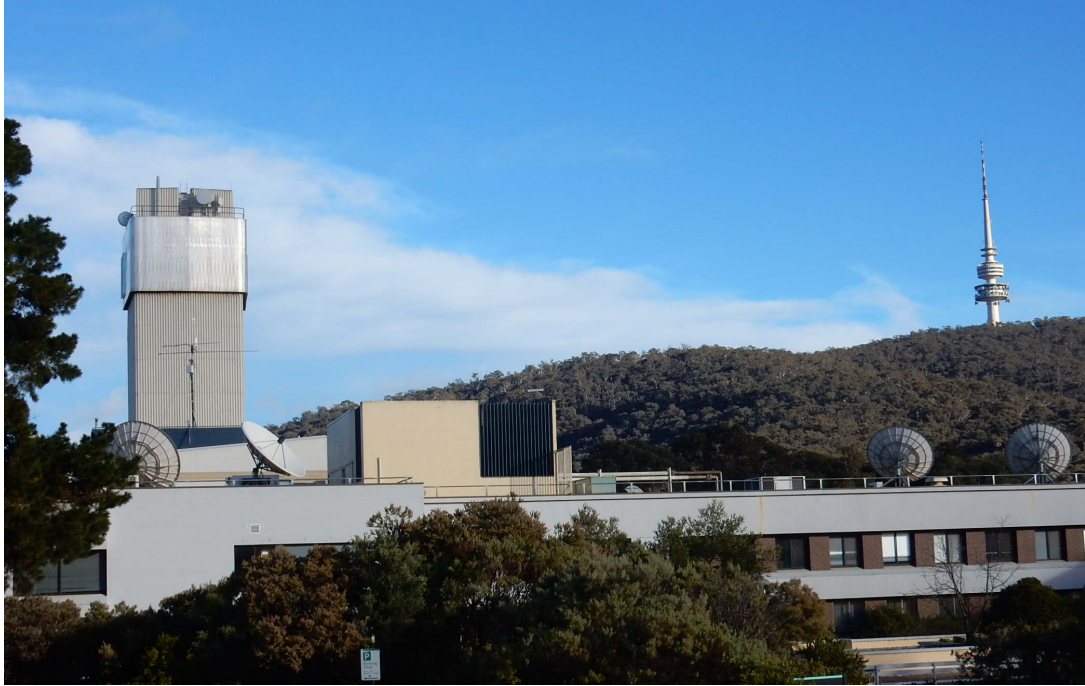
Figure A.2: The ANU ground station antennas (mid left) shows in the local environment
